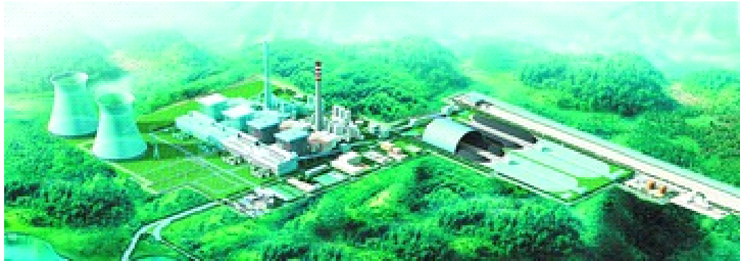
Figure 8.1: Air view of the power station
