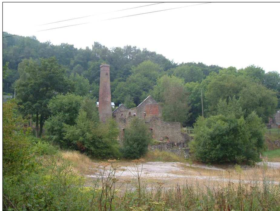
Figure 6-8: A photo of the current state of the compressor house at Snailbeach, Shropshire, UK
