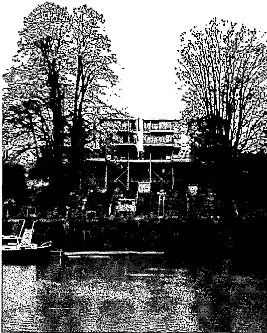
Figure 5: Urban infill housing on a brown-field site in Winchester, 1999. Innovative steel frame construction was required to make this speculative development viable.
