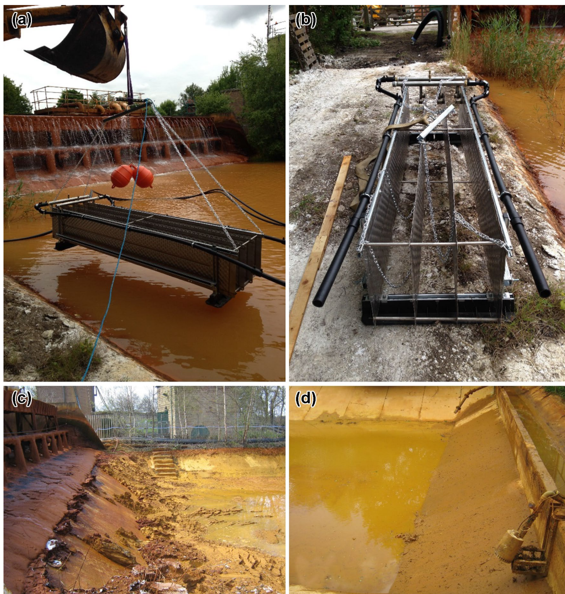
Fig. 9 The Energy Blade™ (b) prior to and (a) during installation in Caphouse No. 1 aeration lagoon; (c) aeration lagoon No. 1 prior to desludging (2013) and (d) aeration lagoon No. 2 following deslud-
