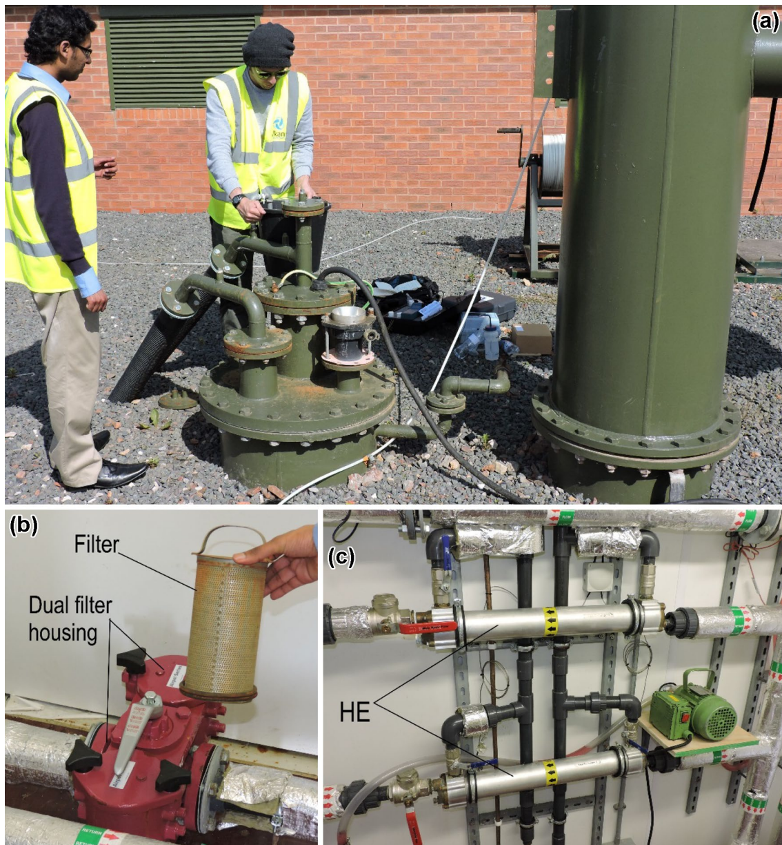
Fig. 7 Markham No. 3 Shaft heat pump system. a Two of the authors (AA and NB) at the shaft top; b mine water filter (relatively unclogged); c shell and tube heat exchangers, marked as HE (pump shown is used for filling and pressurising glycol circuit)
