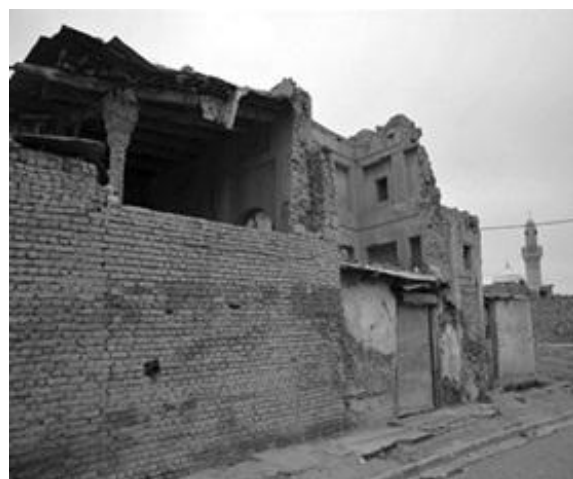
Figure 2: Deterioration of Citadel houses, Erbil (Source: author)
