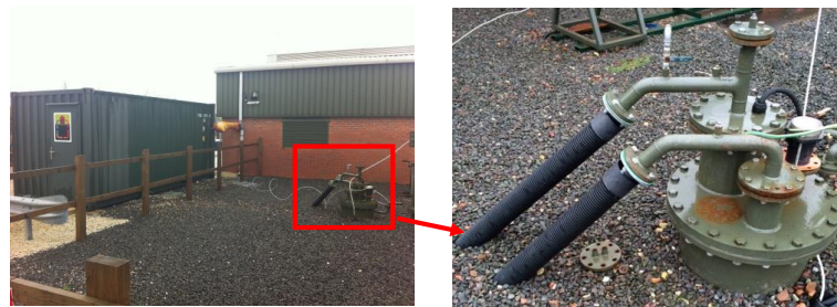
Figure 6.8: Mine water flow and return pipe.
