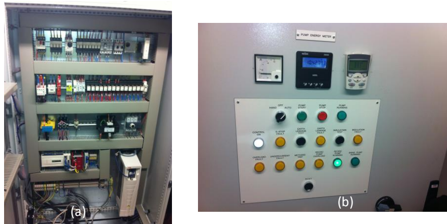
Figure 6.12: Data monitoring and acquisition unit.
