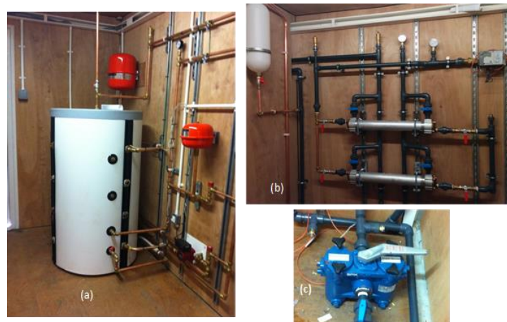
Figure 6.24: Buffer Tank. (b) Prophylactic Shell and Tube Heat Exchanger. (c) Duplex Filter
