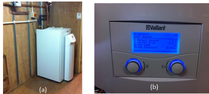
Figure 6.23 : (a). Vaillant GSHP unit. (b) GSHP display screen
