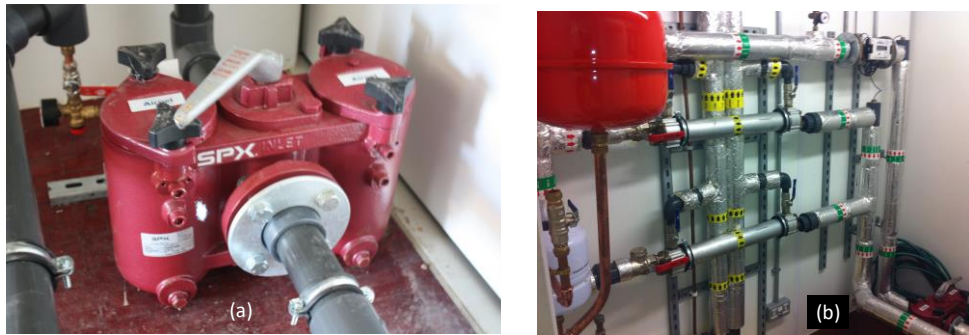
Figure 6.10: (a) Filter.(b) Heat exchanger.
