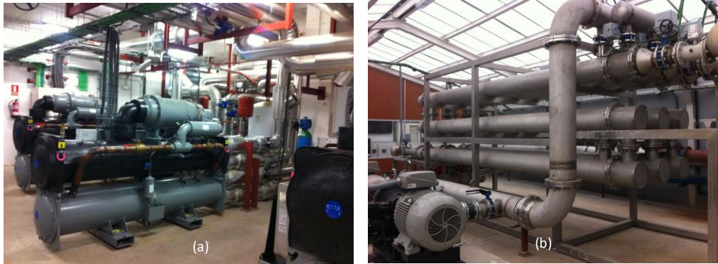
Figure 2.3: (a) GSHP unit at Asturias, Spain. (b) Shell and Tube heat exchanger at Asturias, Spain.
