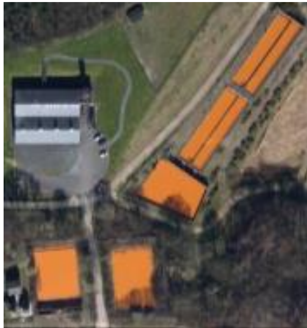
Figure: 6.18: Google map image of the water treatment facility
