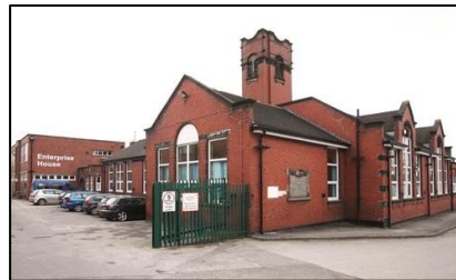
Figure 5.3: The Enterprise building.
