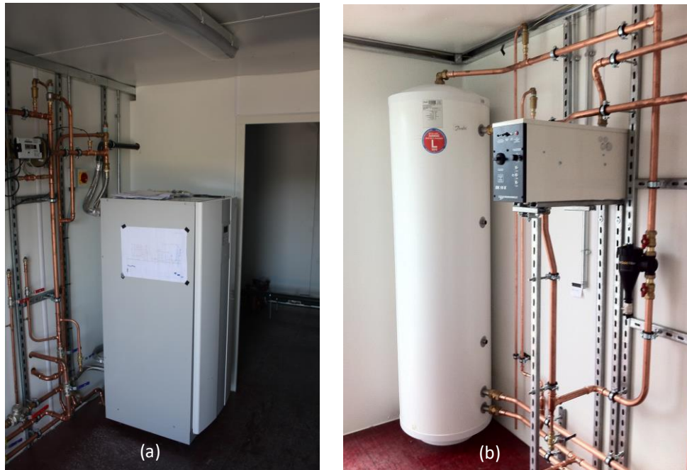
Figure 6.11: (a) Heat pump. (b) Buffer tank.
