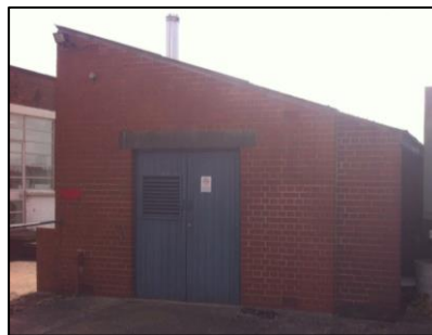
Figure 5.4: The current boiler room
