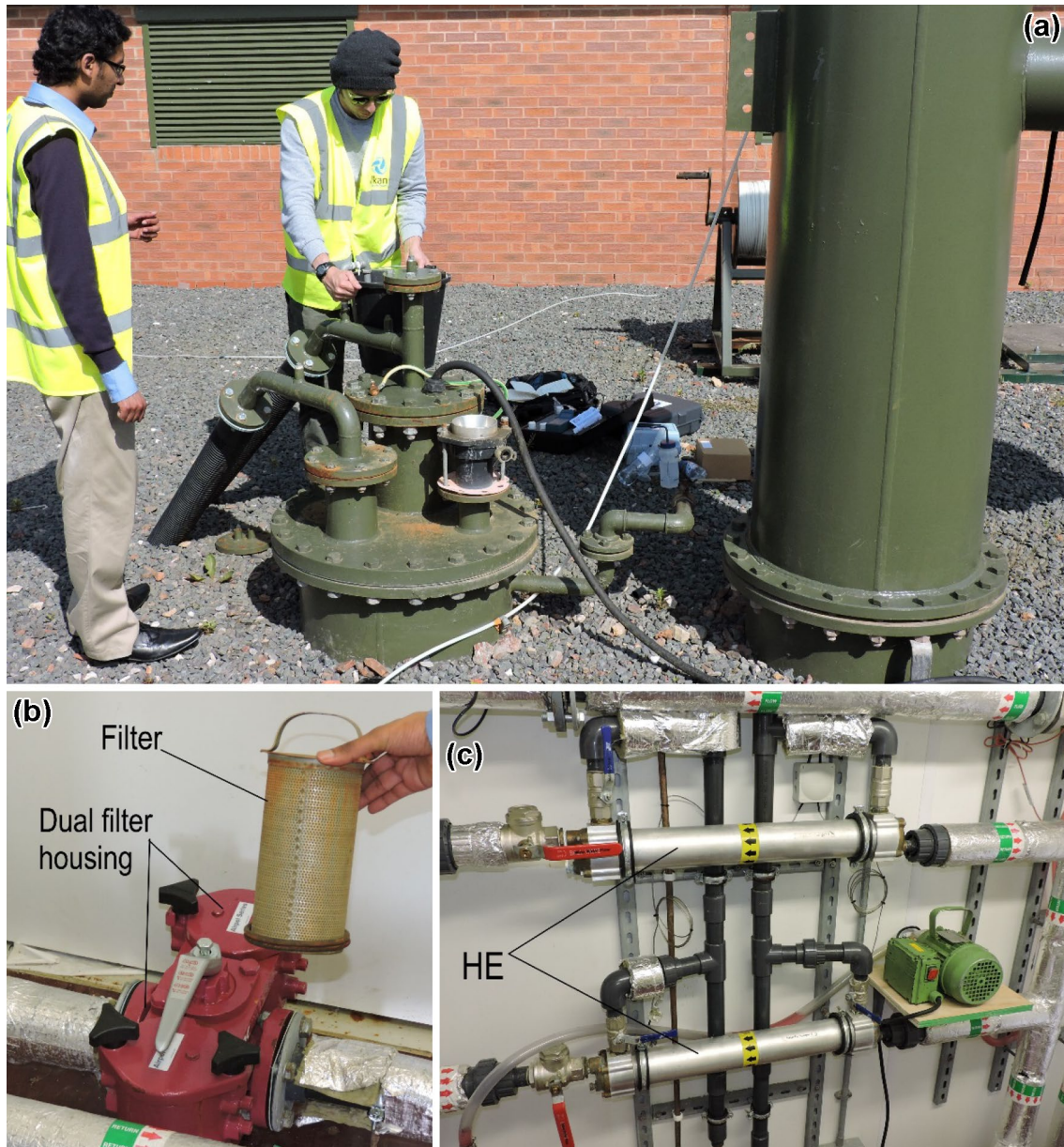
Fig. 7 Markham No. 3 Shaft heat pump system. a Two of the authors (AA and NB) at the shaft top; b mine water filter (relatively unclogged); c shell and tube heat exchangers, marked as HE (pump shown is used for filling and pressurising glycol circuit)
