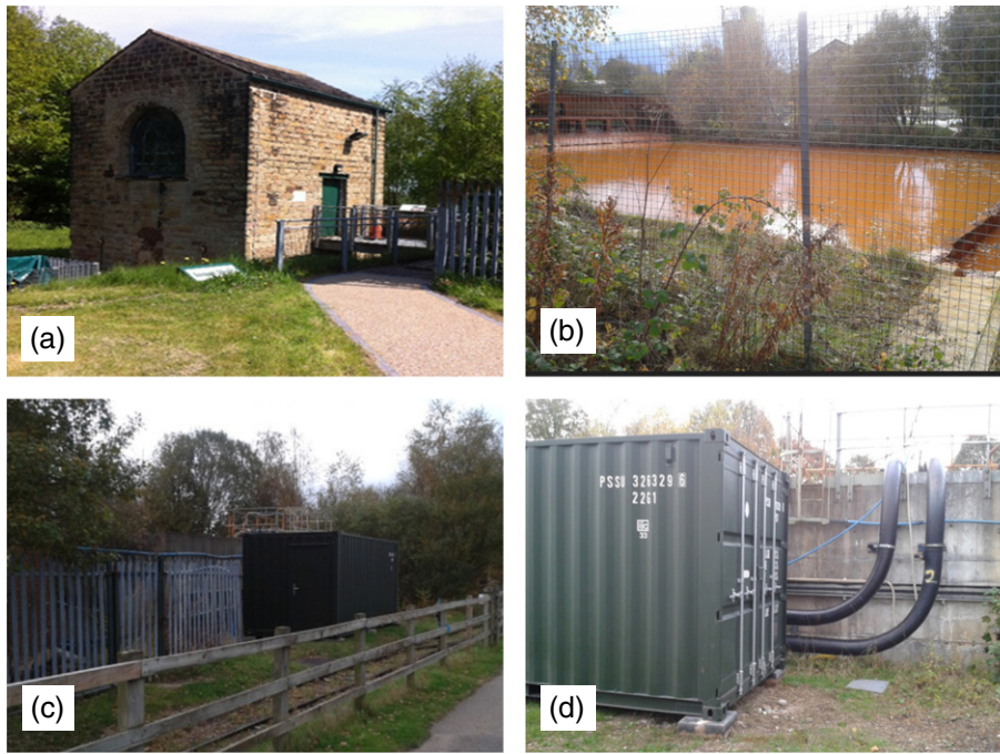
Fig. 3. Main components of the system, Inman shaft building heated by the heat pump (a), the lagoon (b), plant housing container (c) and the container with the main two pipes that pump the water from the coal mine (d).
