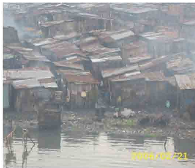
Fig 1: Aerial view of Ajegunle settlement in Lagos, Nigeria. Note the existing housing problem, potential health hazards and organic response to a specific site, potential openness and possibility of relating morphology to cultural variables
