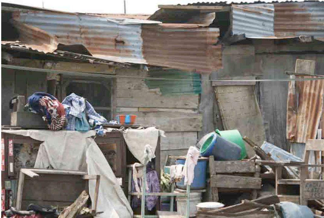
Figure 7.7: FRONT AREA OF A RESIDENTIAL BUILDING (Photograph by Olusegun Oluwole).
