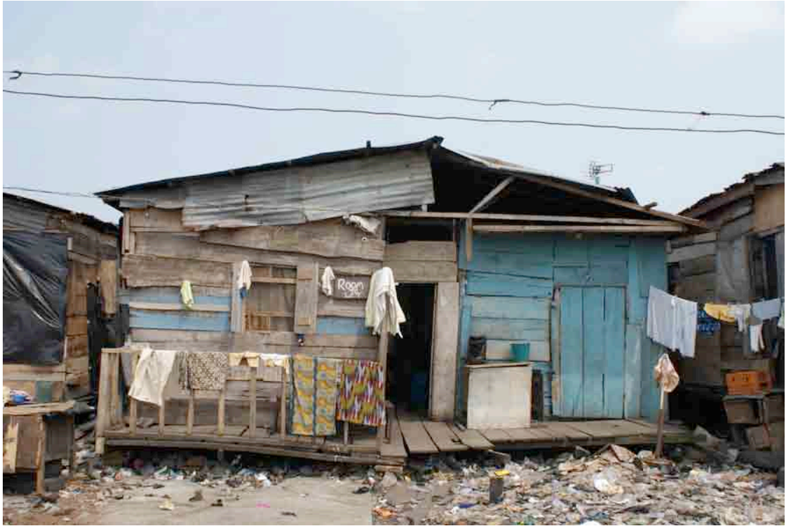
Figure 7.10: FRONT ELEVATION OF A RESIDENTIAL BUILDING IN THE COMMUNITY (Photograph by Olusegun Oluwole).
