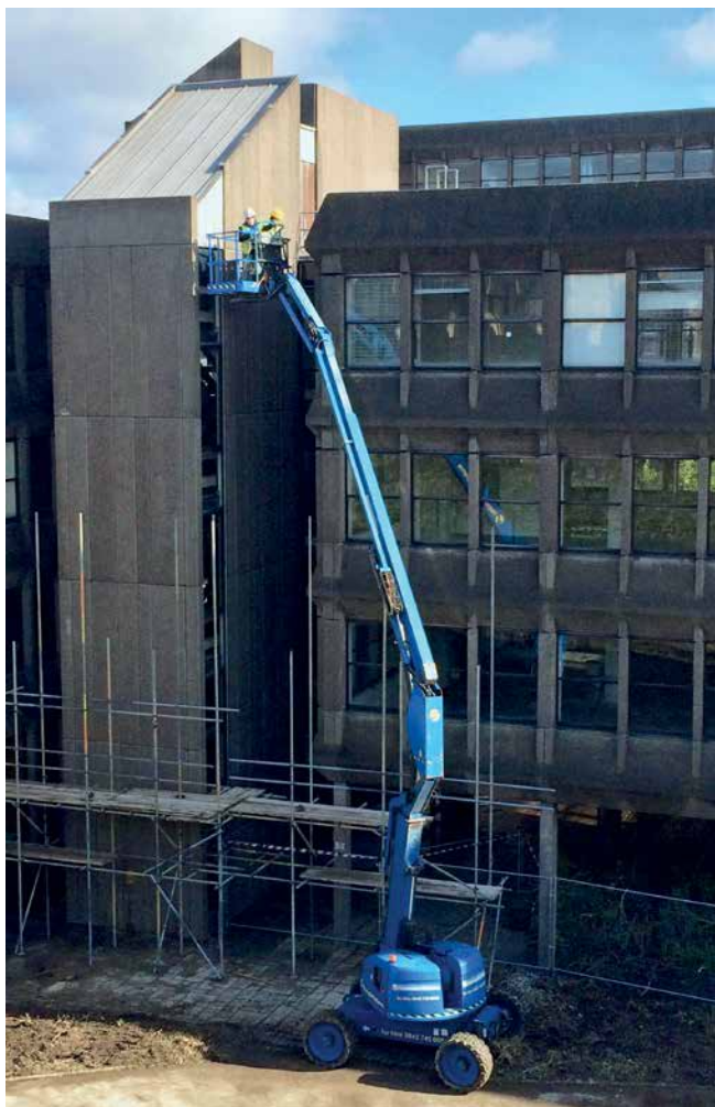
Figure 2. Surveys may need to support both planning requirements and the needs of protected species licensing. Here, bat roosts are being inspected and excluded following a number of detailed surveys and grant of a mitigation licence.
