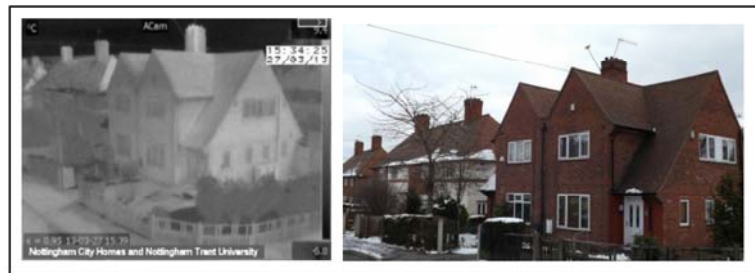
Figure 2 : An Example of the infrared results obtained for the group of buildings.
