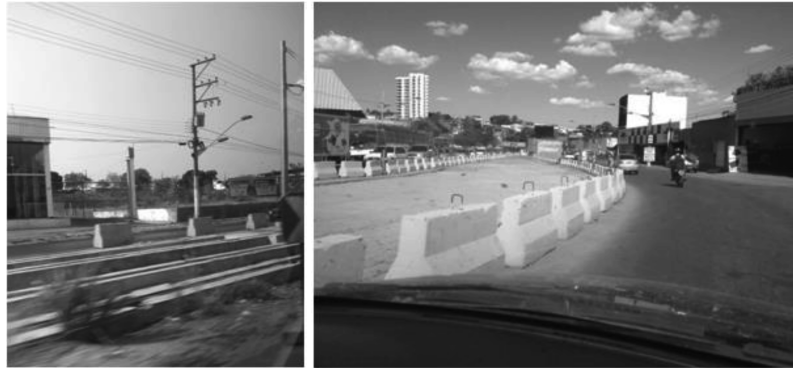
Figure 2. The VLT railway in Cuiabá, an unfinished infrastructure program associated with the 2014 World Cup (author's own photographs).
