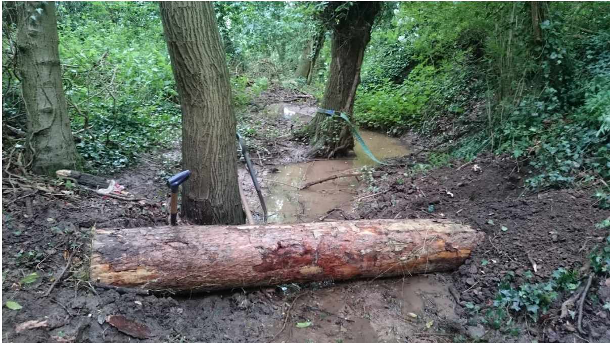
Figure 5.16 Construction of LWD dam 2 within the Springfield Dumble (view from upstream).
