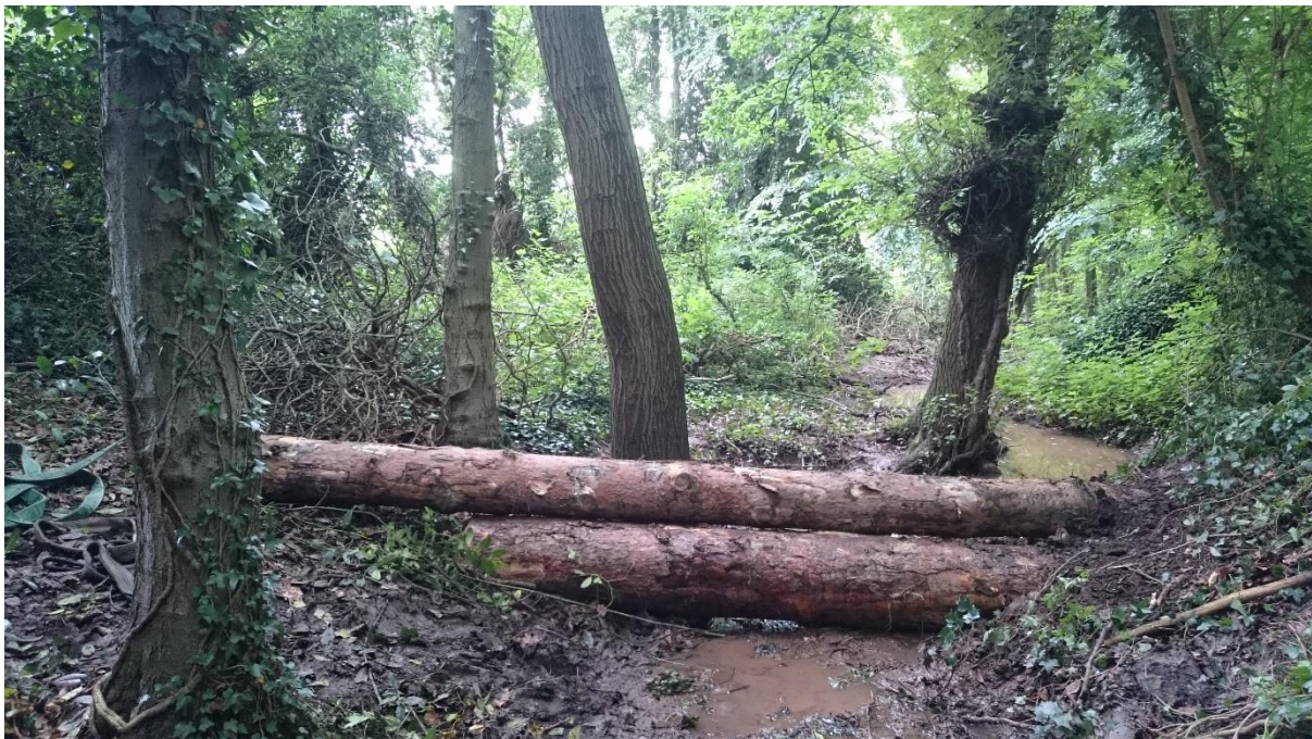
Figure 5.17 Completed LWD dam 2 within the Springfield Dumble, showing a gap to allow the passage of low flows (view from upstream).
