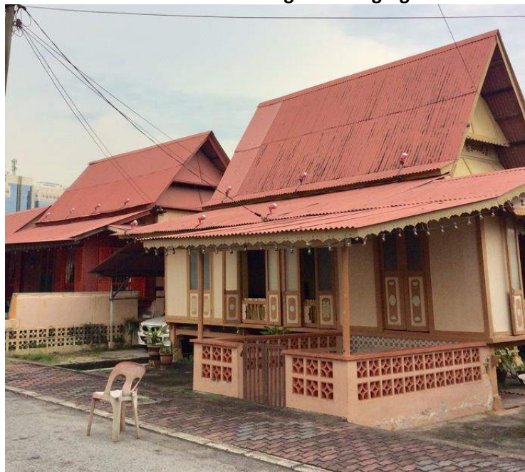
Figure 44: A traditional house in Morten village showing signs of deterioration
