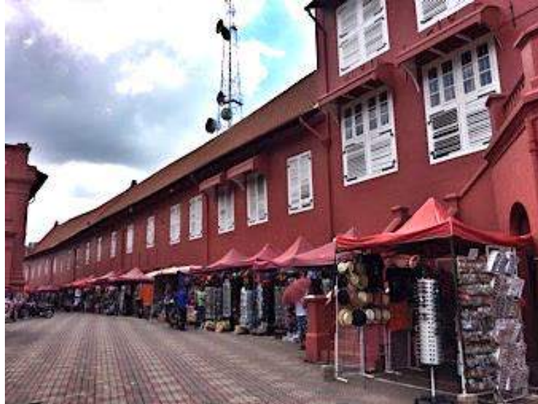
Figure 52: A row of stalls damaging the image of historic Stadthuys buildings
