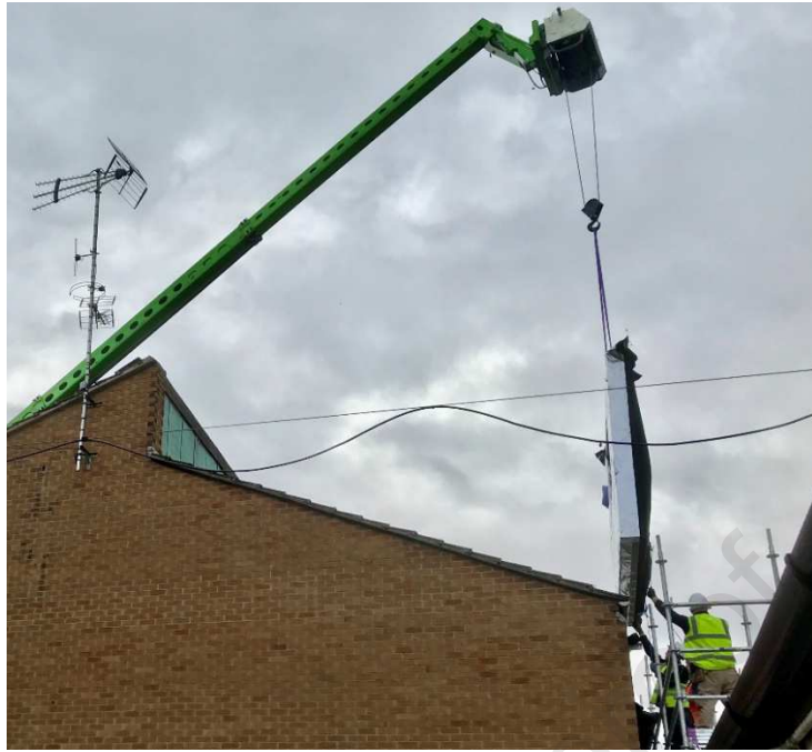
Figure 5. Installation of a prefabricated façade module
