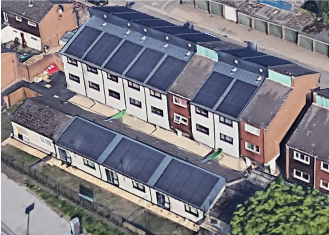
Figure 4. Satellite view of the cluster after the refurbishment
