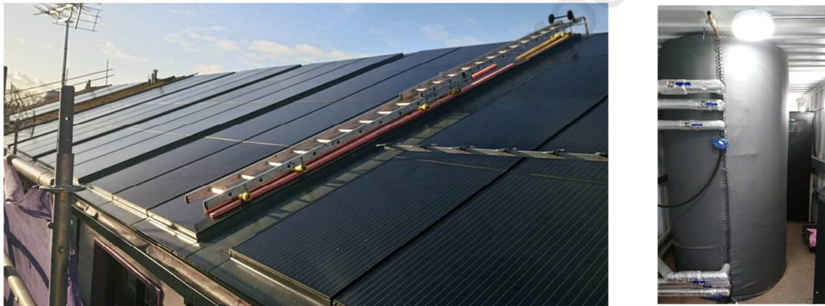
Figure 7. Photovoltaic plant and TES
