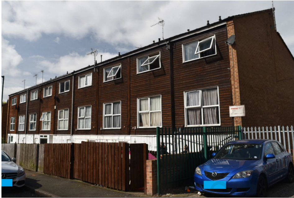
Figure 3. Back of the building before the refurbishment
