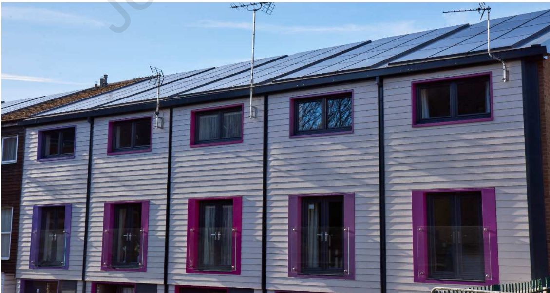
Figure 6. Back façade of the building after the retrofitting
