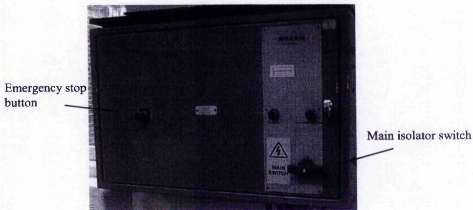
Figure 9 Main power switch for running the machine
