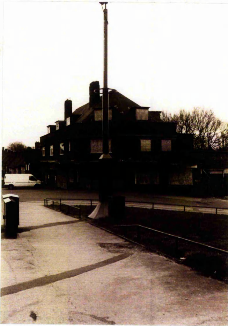
Plate 1 Showing the burnt out Boarded-up shops close to Henry Whipple School. In the foreground is one of the security cameras installed throughout the estate
