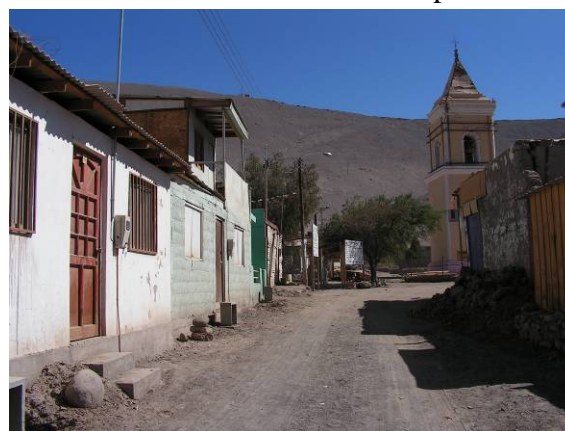
Figure 1: View of Vigueras street. San Lorenzo de Tarapacá, Chile. 2006.
