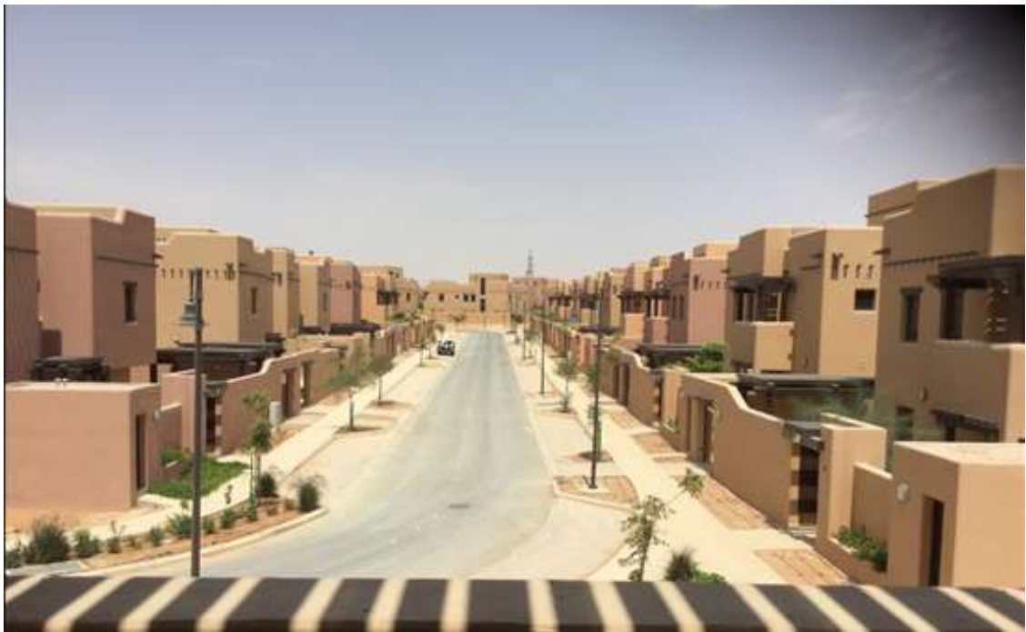
Figure 6.12: View of the residential complex (Source: Saudi Projects, 2017)
