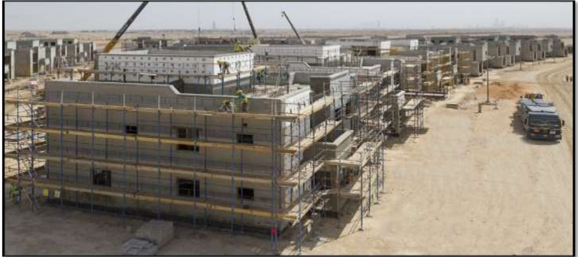
Figure 6.11: External finishing of insulators (Source: DMC, 2019)
