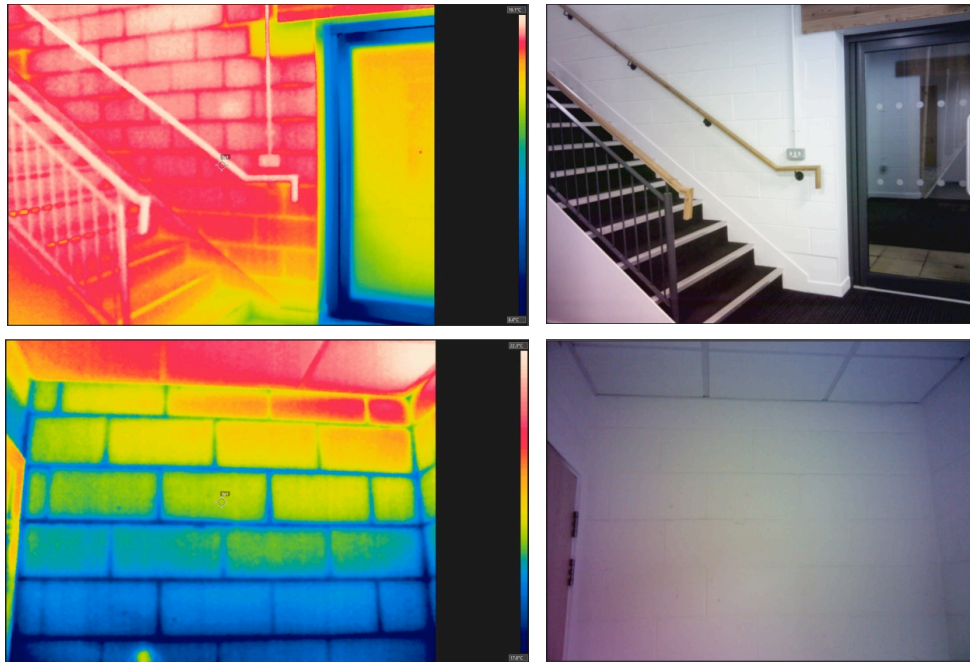
Figure 5-17: Heat losses and gains from the entrance with digital images (right)
