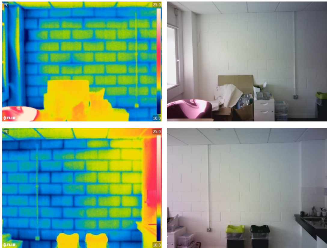
Figure B-0-2: Thermal images and digital images of the external wall in main-lounge
