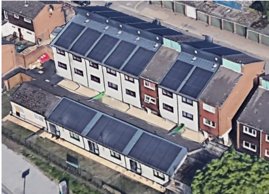
Figure 8: Terraced 3-Bedroom Homes and Bungalows After Retrofit
