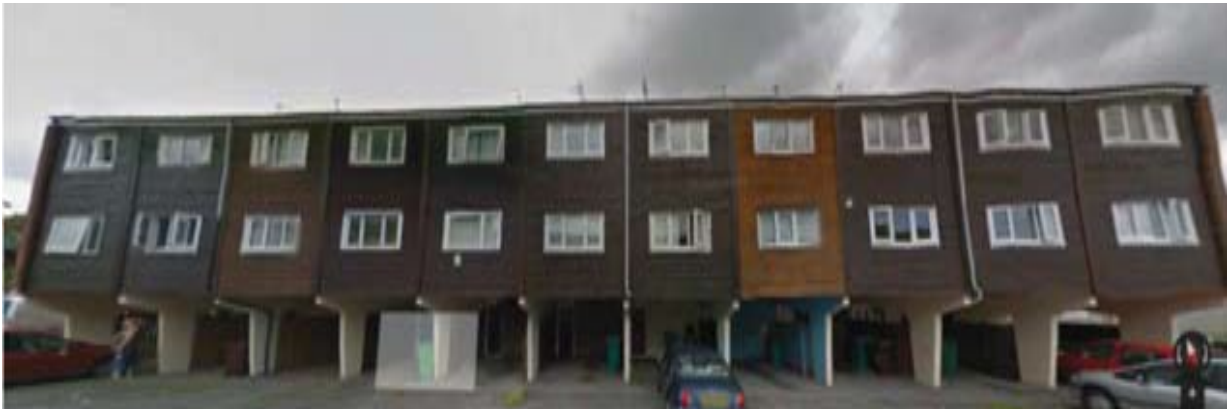
Figure 7: Terraced 3-Bedroom Homes Before Retrofit
