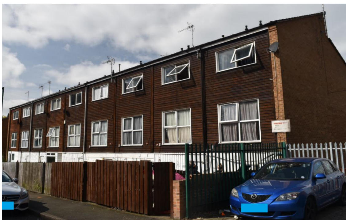
Figure 5.6. Back of the building before the refurbishment
