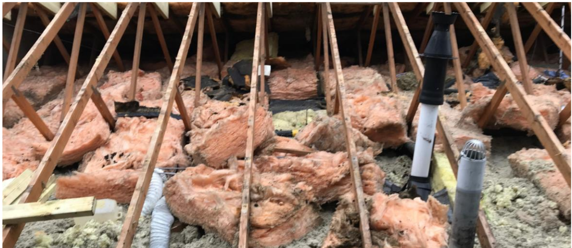
Figure 5.10 Loft insulation in one of the bungalows
