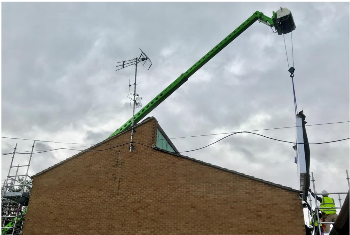
Figure 5.12. Installation of a prefabricated façade module
