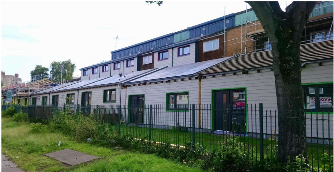
Figure 5.11 Case study after the refurbishment intervention
