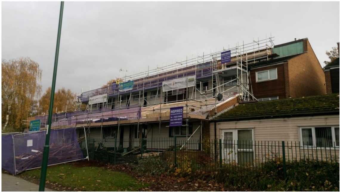
Figure 5.3 Case study during the refurbishment work
