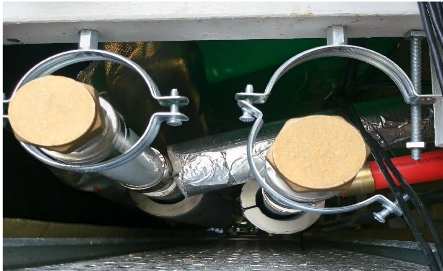
Figure 5.14 Piping before being covered with the new insulation layer
