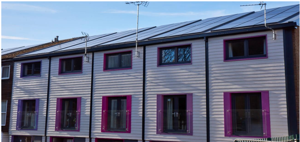
Figure 5.13. Back façade of the building after the retrofitting
