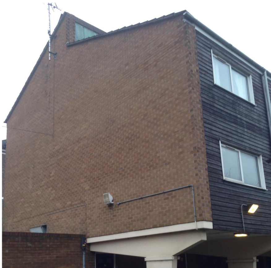
Figure 5.5 End terrace wall pre-refurbishment
