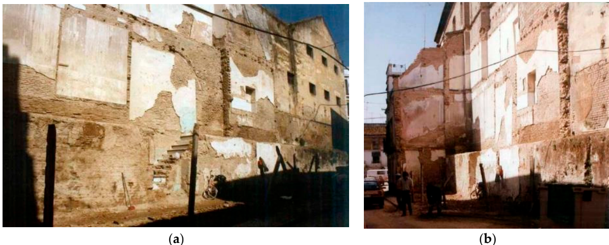
Figure 23. Photographs of demolished houses near Puerta Real, at 3 Goles Street, next to the San Laureano building and remains of the city wall, 1990. Urban Planning Management, Seville City Council [available online: https://www.urbanismosevilla.org/areas/proyectos-y-obras/publicaciones/fototeca/muralla (accessed on 15 April 2023)]: (a) View to the north; (b) View to the south.
