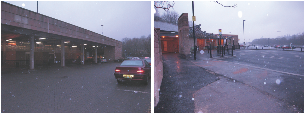
Figure 5.1 Old Bus station (Bakewell Road) and New Bus station (Cawdor Quarry)
