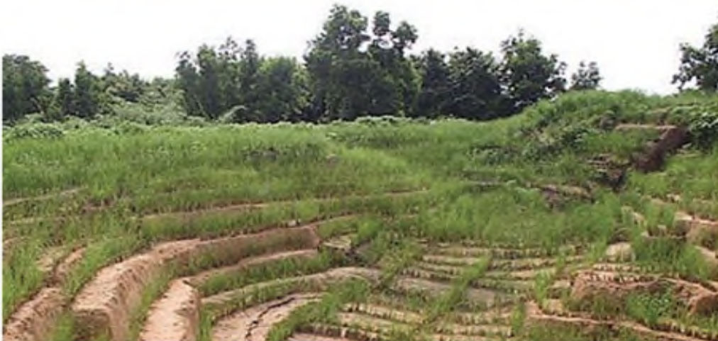
Figure 2.10: A Vetiver grass system is being used in the Democratic Republic of the Congo for gully control in urban areas and for highway stabilization. These gullies are a major problem in this area and other West African countries (top); the same slope now has improved drainage, and the slope has been planted in Vetiver grass (middle); this planting of Vetiver grass is about three months old (bottom) (Highland and Bobrowsky, 2008)
