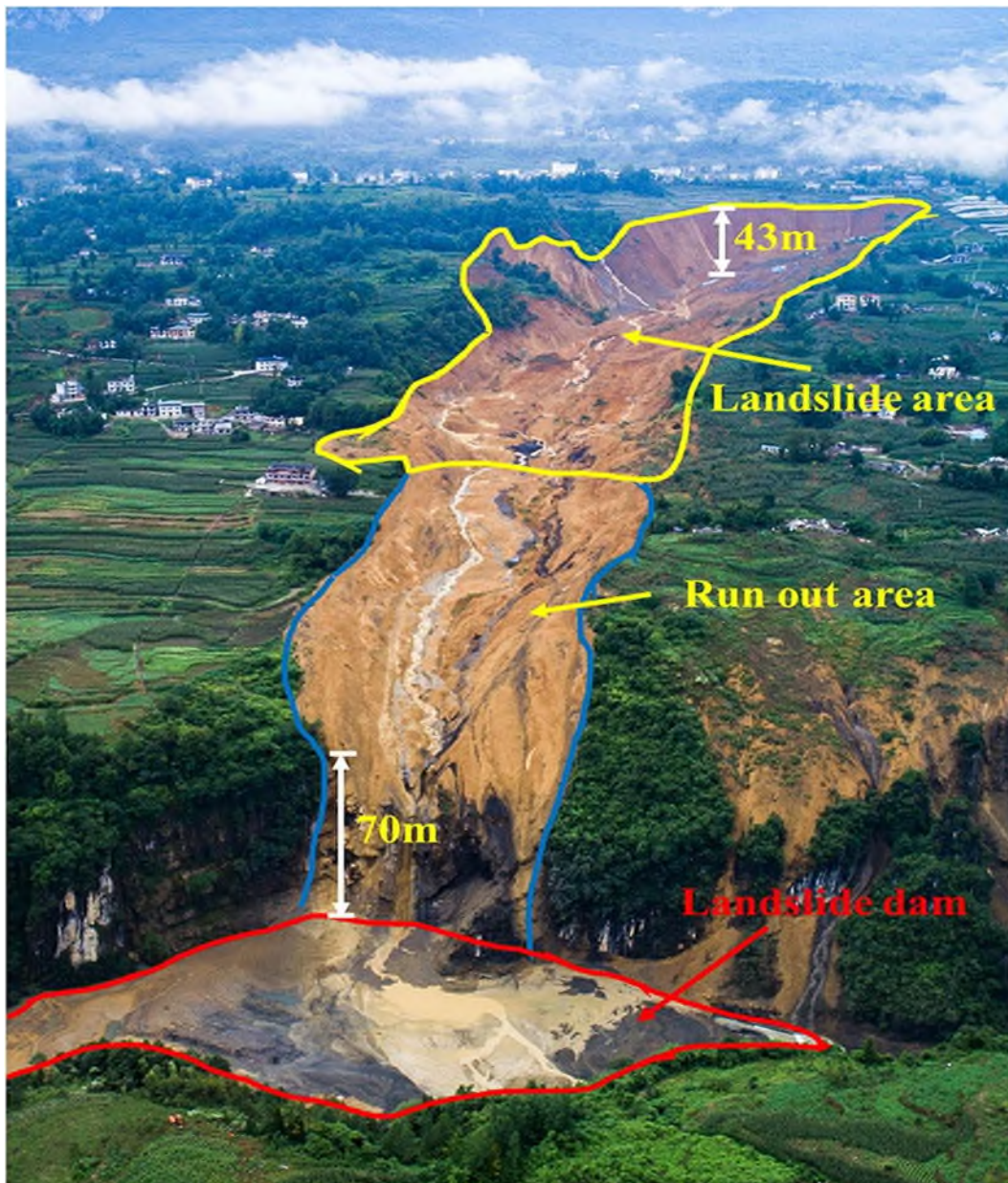
Figure 1.2: Shaziba Town Landslide and formation of landslide Dam (Tengfei et al. 2012)
