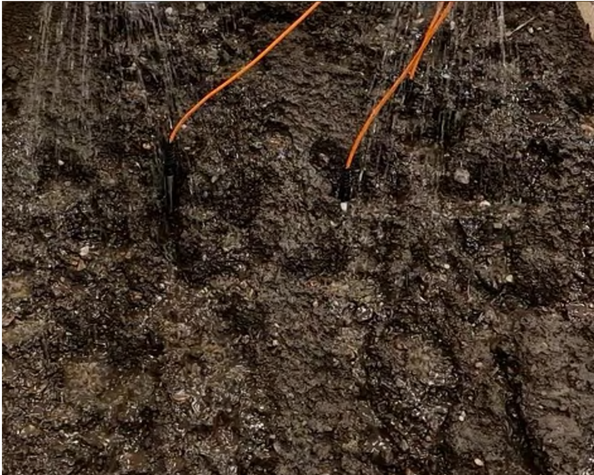
Figure 5.18: To surface of stabilised slope after failure
