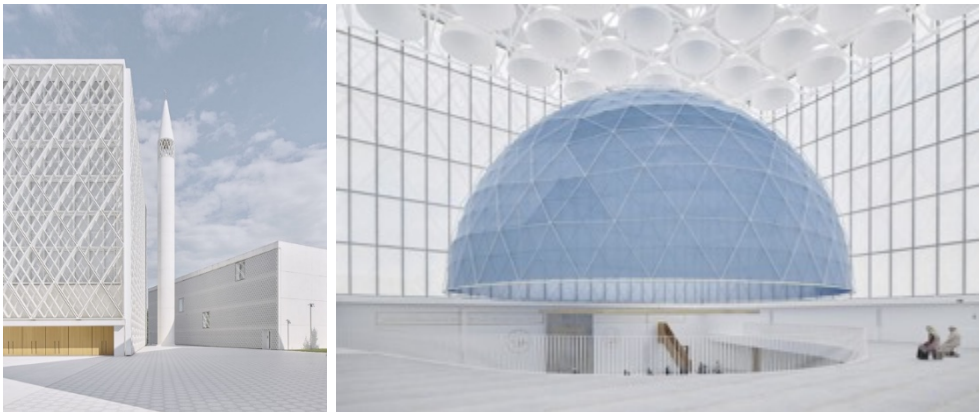
Figure 5-32 The minaret of Ljubljana Mosque standing between the mosque and the educational building (left) The small cupolas above the suspended main blue dome (right). Photographs by David Schreyer (The Architectural Review)
