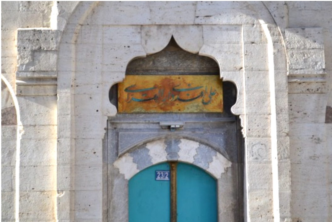
Figure 4-13 The Kadi Haci Ali Efendi Darul Kurrasi, a Qur'an Madrasah built in 1428, it was closed after the establishment of the republic and turned into health museum, town hall supplement, library and police station, among other things (Author 2021)
