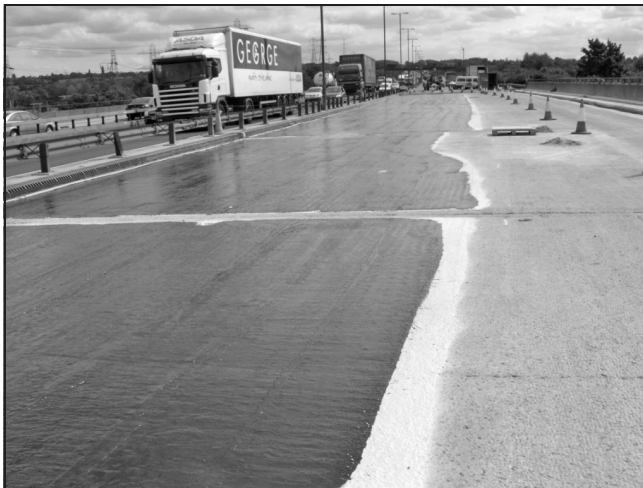
Figure 1. Preparation for surfacing on the northbound carriageway for P2
