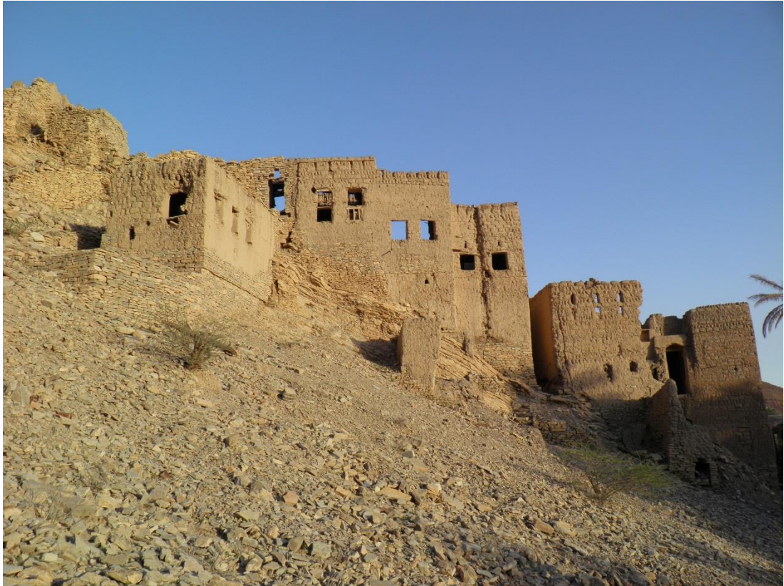
Figure 42: The gradual reduction in the terrace stone foundation height in the less steeper levels of the slope.
