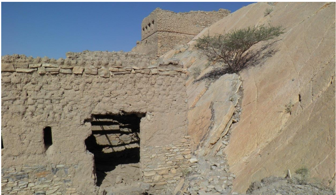
Plate 13: Phase-2 of Ḥarāt as-Saybānī, a. the tower and the boundary wall constructed behind it, b. natural rock formation used as an anchor for the structure foundation, c. the large rock layer forming the south edge of phase-2.
