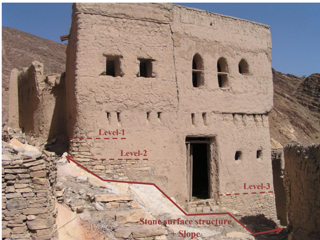
Figure 43: The varying height levels of the stone foundation walls influenced by the steepness of the slope and the advanced construction technique of the dwellings in Ḥarāt as-Saybānī.
