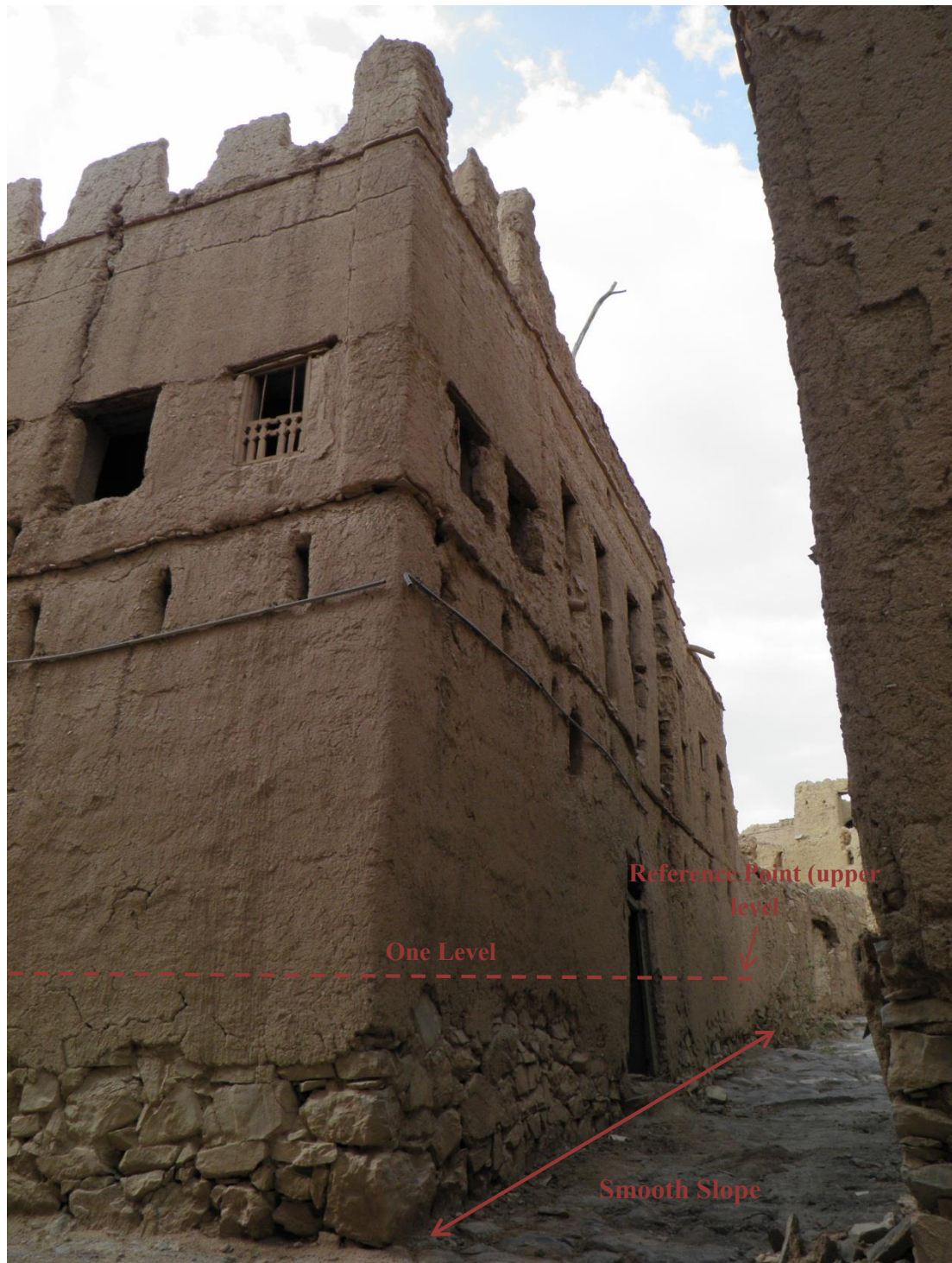
Figure 44: The stone foundation walls in the dwellings of Ḥarāt al-Wiṣṭā maintain the same height level with reference to the height of the upper stone foundation in the upper level.
