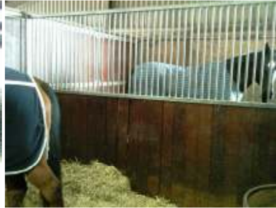
Figure 1.2. Stable type offering visual contact with neighbouring horse via internal bars.
