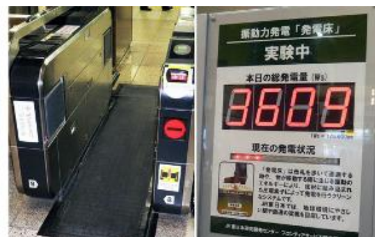
Fig. 3. Piezoelectric system in Tokyo Subways [2]
