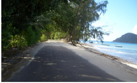
Figure 5.3.11 Road encroachment at Machabée
