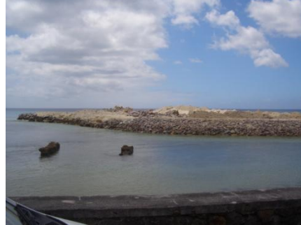
Figure 5.3.19 New groins Mahé
