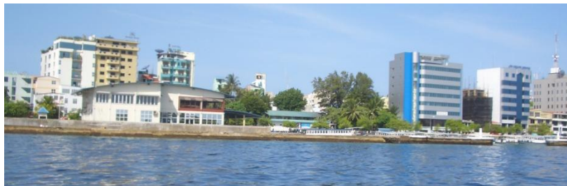
Figure 5.2.8 View of wall at Malé from Malé International Airport
