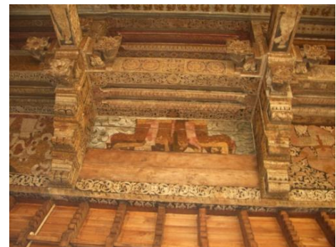
Figure 5.1.12 Anuradhapura, wood carving in need of restoration
