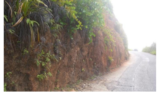
Figure 5.3.12 Landslip on Praslin
