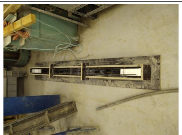
Figure 2: Beam E- Preparation to cast the beam with two polystyrene blocks.
