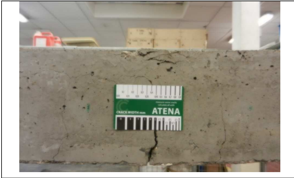
Figure 6.7: Beam C - mid span zone at the final damage state-photograph.
