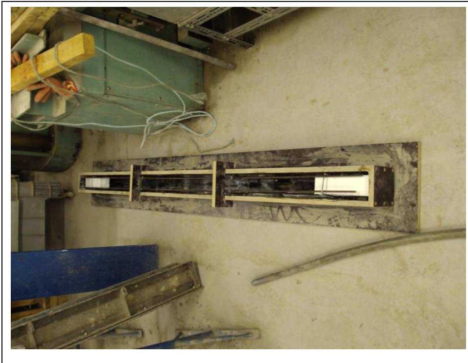
Figure 6.8: Beam E- Preparation to cast the beam with two polystyrene blocks.
