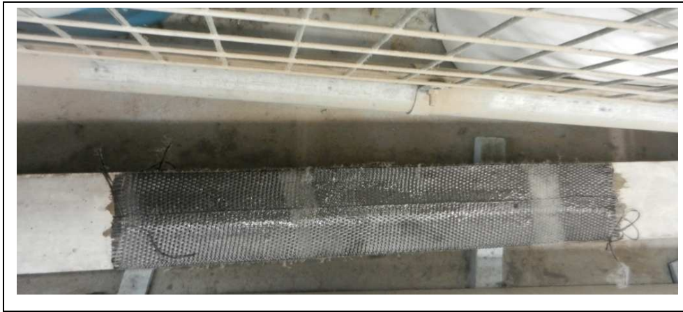
Figure 6.3: Beam A - strengthening with CFRP layers-photograph.
