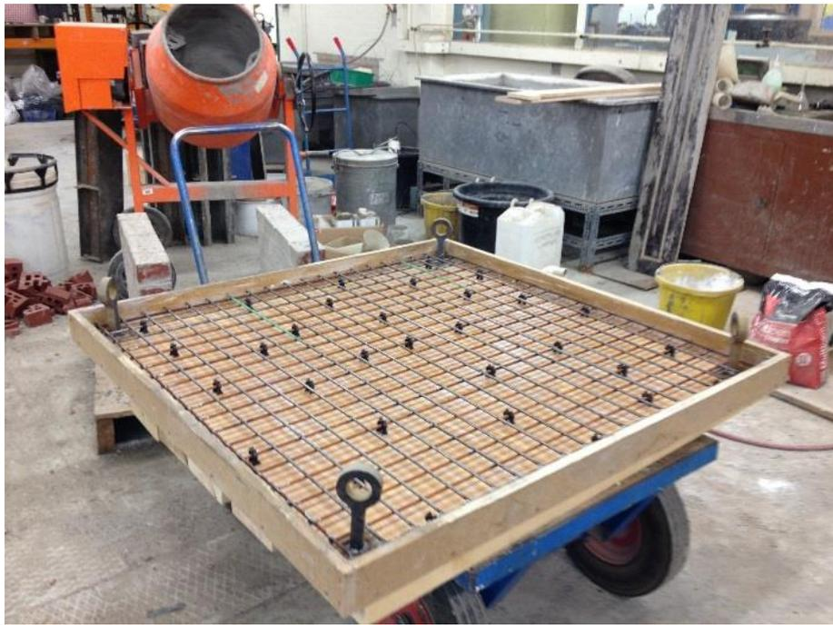
**Figure A. 2:** Placement of steel reinforcing mesh.
