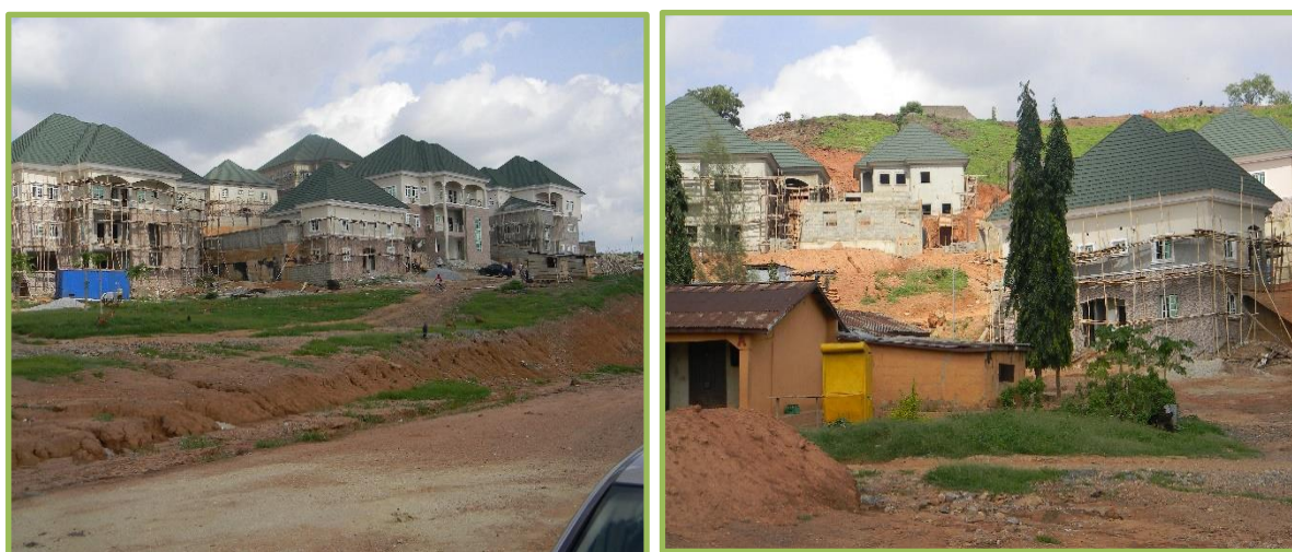
Figure 6.23: The Transformed Kuruduma Neighborhood with New Residential Layout in Developed by Private Developers in Replacement of the Indigenous Buildings. Source: (Own Photograph, May 2013).
