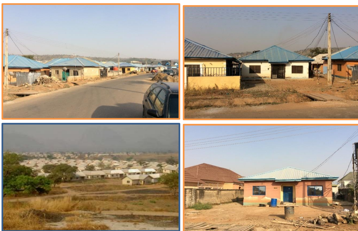
Figure 6.9: Abuja Government Compensation and Resettlement Housing Scheme ( Photograph: Segun Ogunsola, 2015 ).
