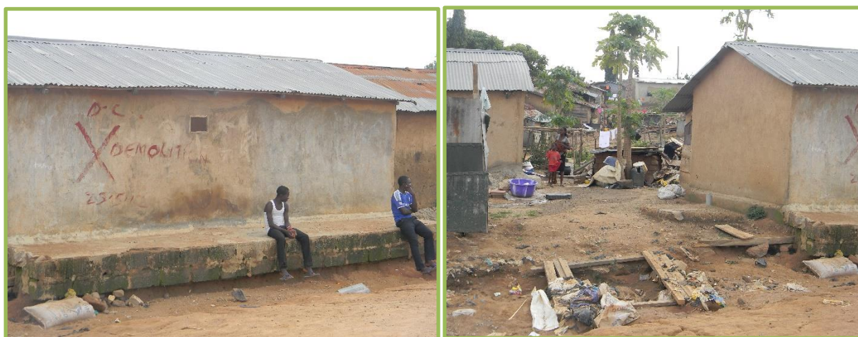
Figure 6.22: The Kuruduma Residents Awaiting the Bulldozers as their Residential buildings are Marked for Demolition by the Abuja Government. ( Own Photograph, May 2016 ).
