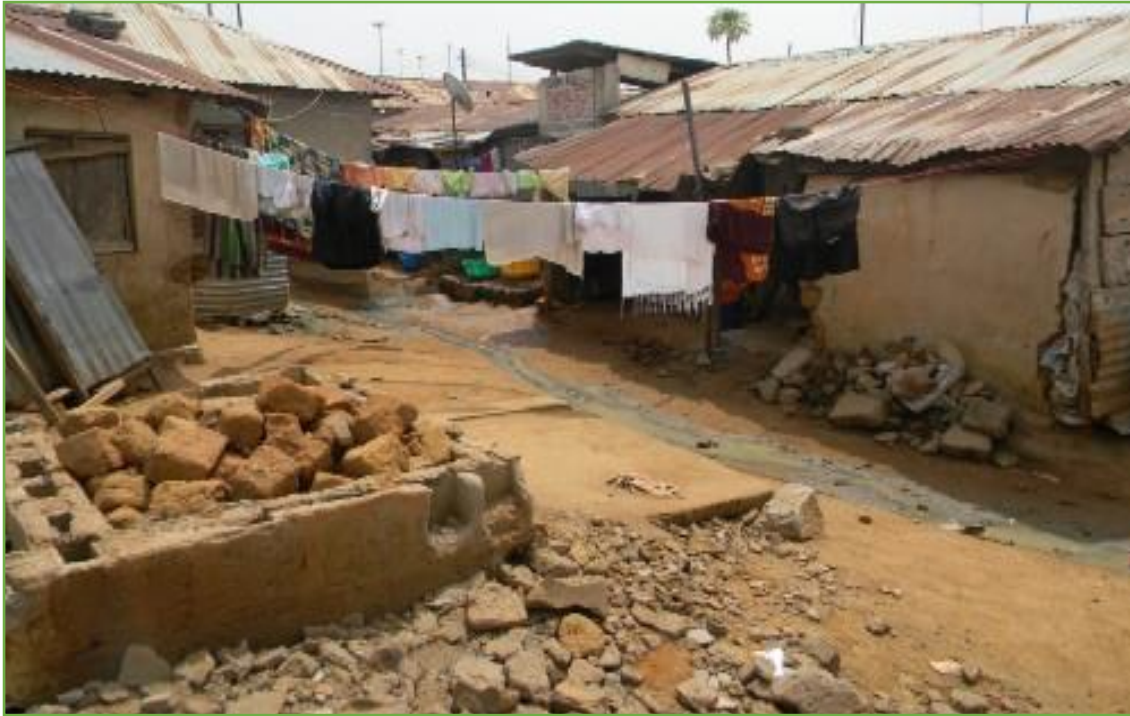
Figure 6.17: The Dilapidating State of the Inner Part of Dutse-Bwari Community has been shown by a Resident During the Empirical Process. ( Own Photograph, May 2013 ).
