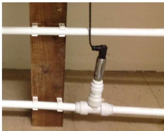
Figure 4.24: The upstream pressure sensor in situ
