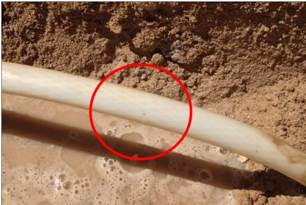
Figure 6.17: The leak hole after cleaning
