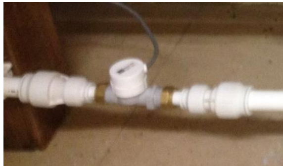
Figure 4.30: The upstream flowmeter in situ
