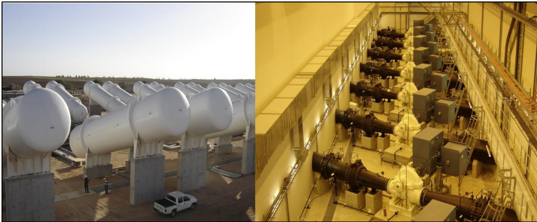
Figure G-3: Pump stations and Surge Vessels
