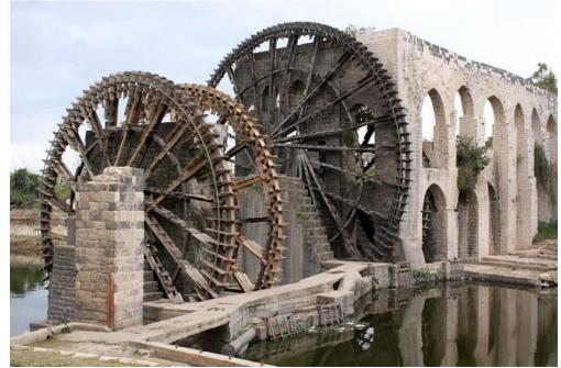
**Figure 1.10:** The large Norias, wooden waterwheels built by the Mamluks, taken by Anon **Source:** Syrian Researchers, 2000
