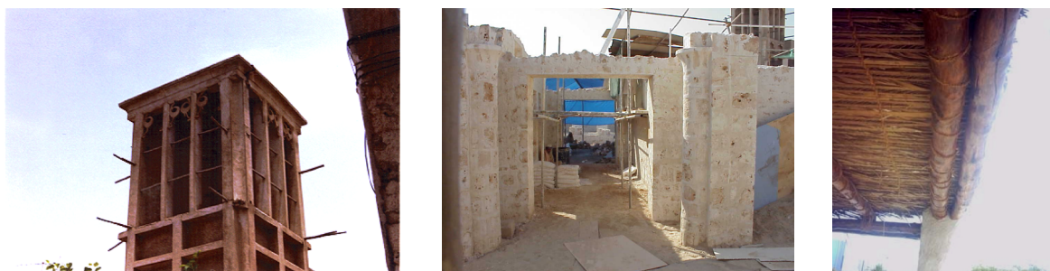
Fig 7. Al-Bastakiyah Houses: Environmental and material tectonics for weather-related performance.
