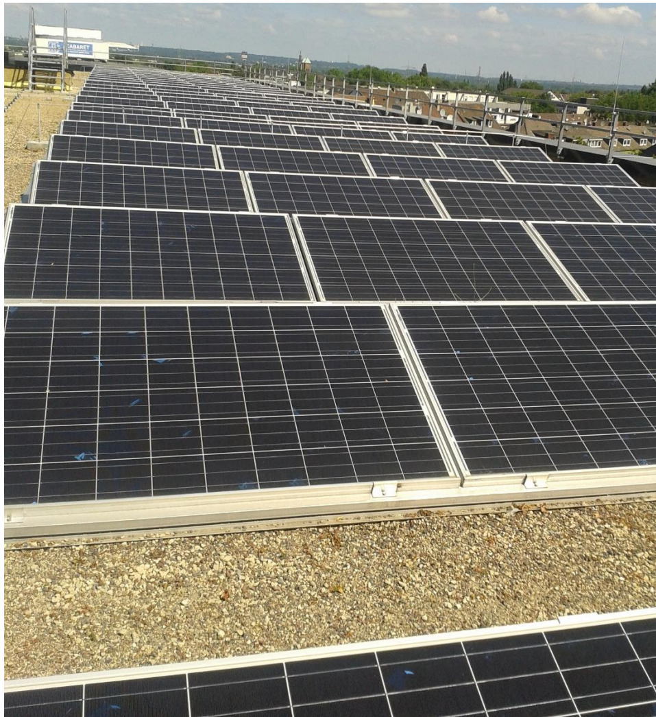
Figure 5.8: Photovoltaic panels on the roof of Hans-Sachs-Haus (photograph taken in July 2013)
