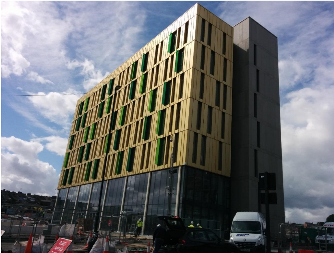
Figure 5.3: The Core Building, Science Central (photograph taken in August 2014)
