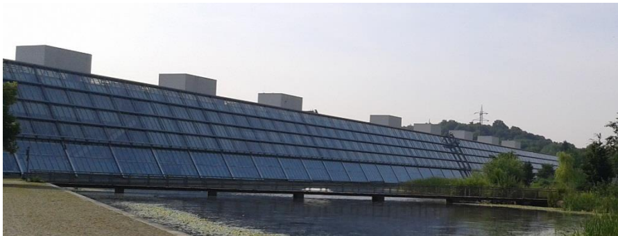
Figure 4.4: The PV panels on Gelsenkirchen's science park (Wissenschaftspark, photograph taken in July 2013)
