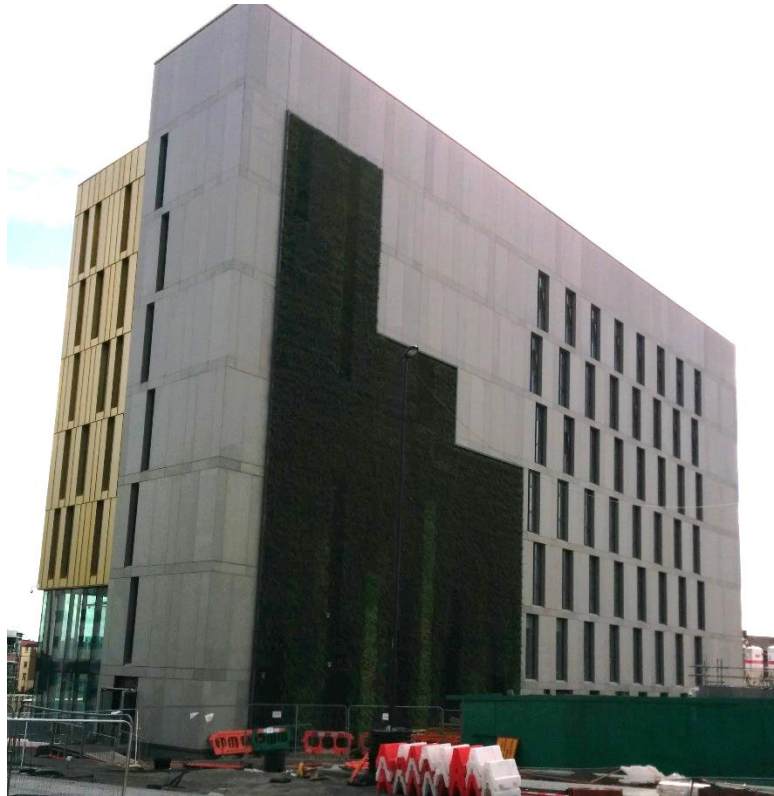
Figure 5.9: The 'living wall' on the side of the Core Building (photograph taken in August 2014)
