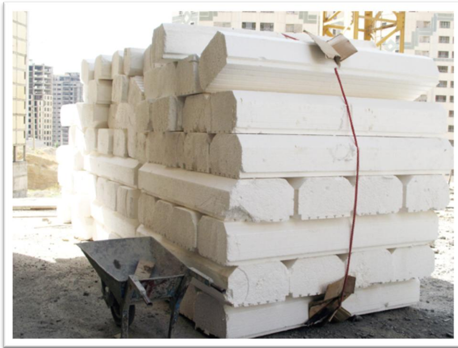
Photo 21: Straps damage the foam floor sections
