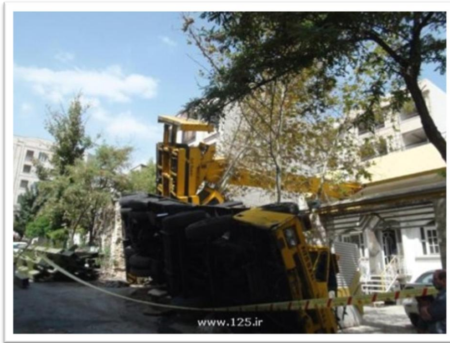
Photo 25: Collapsed mobile crane (Tehran-Fire-Station, 2010)
