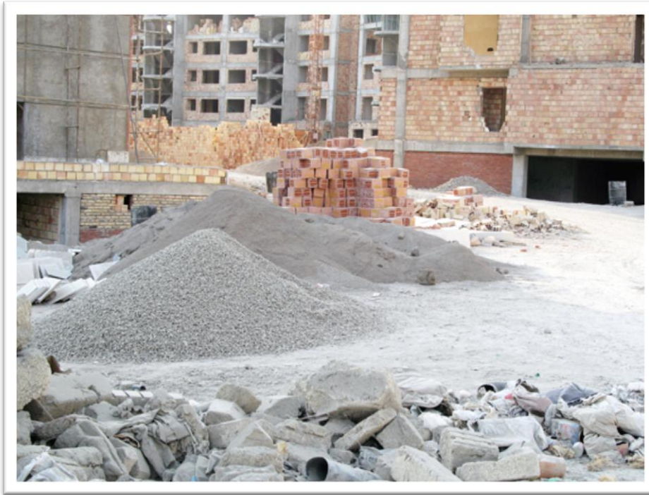
Photo 36: Gravel, sand, bricks and blocks are stored in the outdoor space
