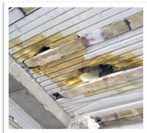
Photo 6: Foam roof sections damaged by heat
