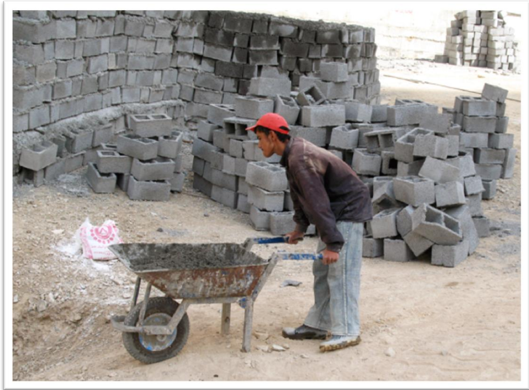
Photo 28: Materials temporarily stored near the building to be handled to the point of use gradually by means such as a wheelbarrow
