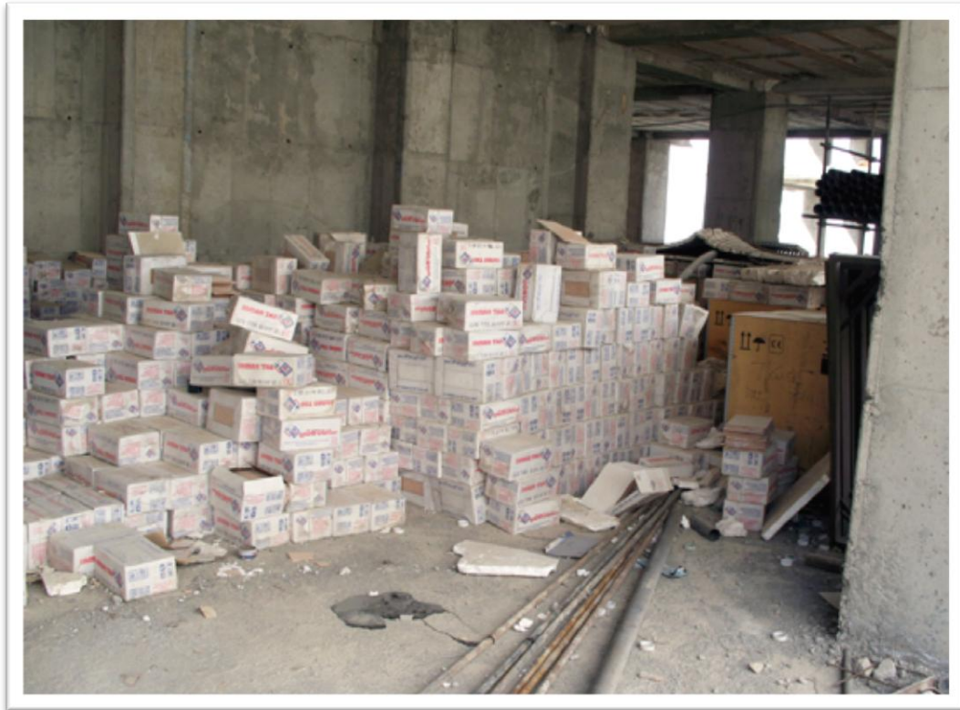
Photo 33: Disorganised onsite warehouse
