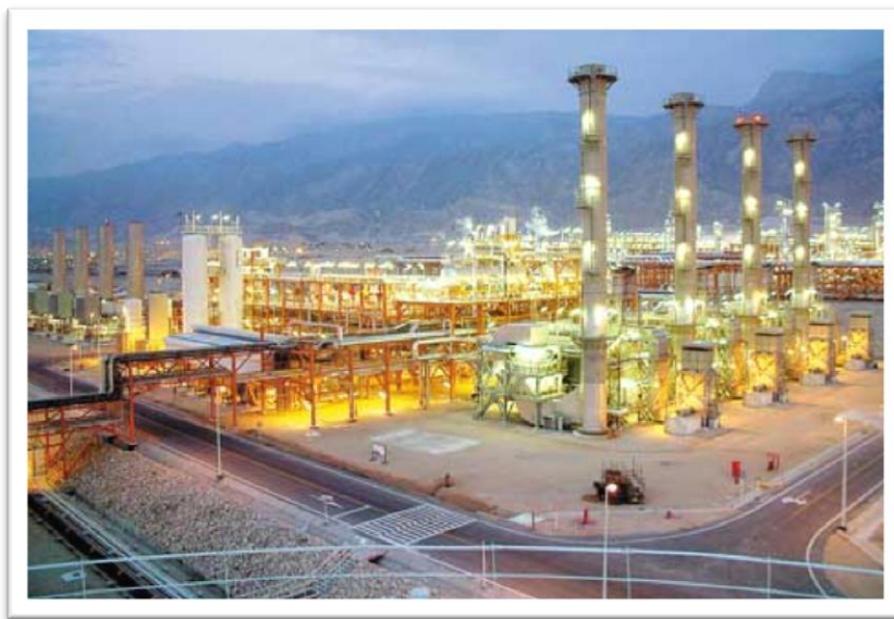
Photo 1: South Pars phases six, seven and eight (JamejamNews, 2008)
