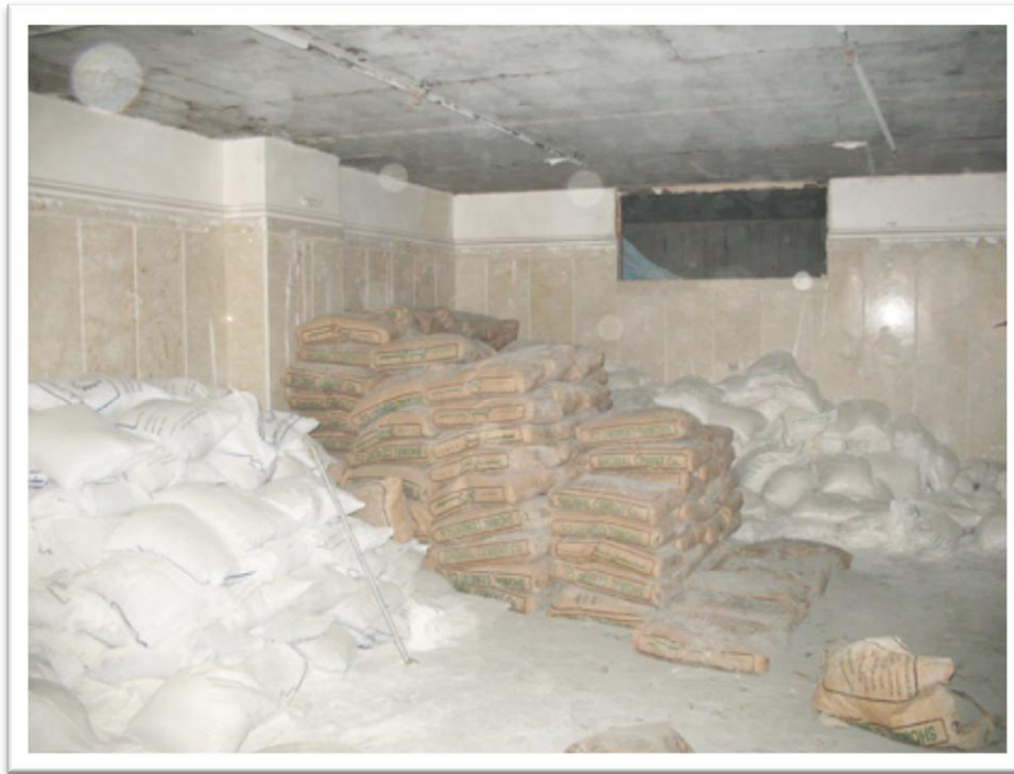
Photo 37: Cement and gypsum powder bags stored in the basement of a building
