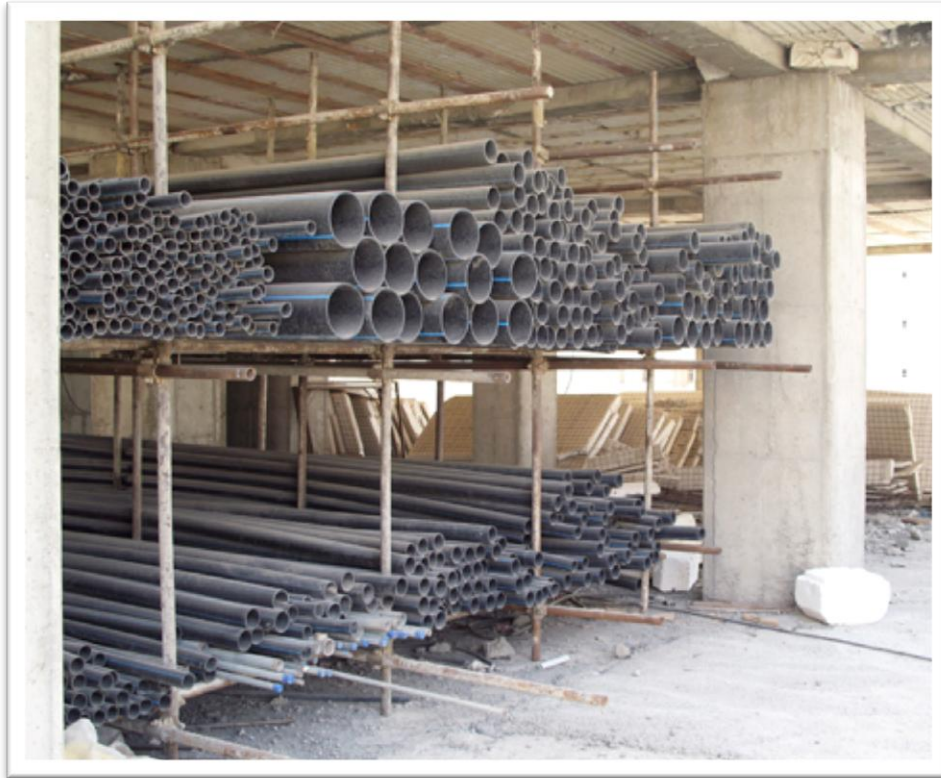
Photo 34: PVC pipes are properly stored and categorised by size in an indoor storage space
