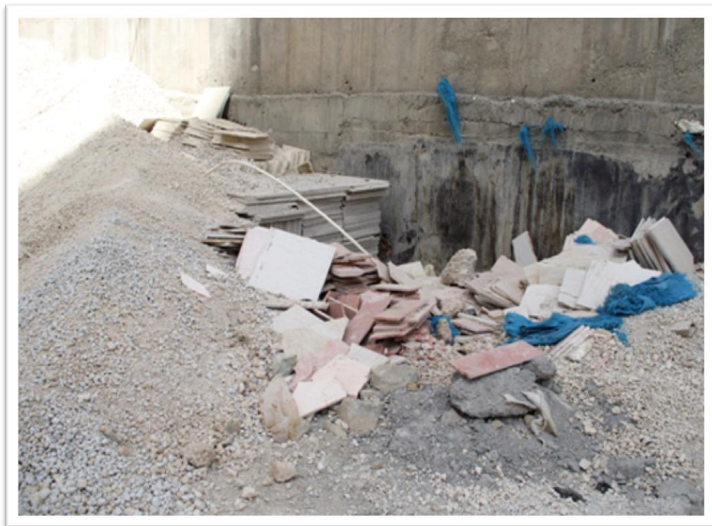
Photo 32: Dirty site owing to poor warehousing practice
