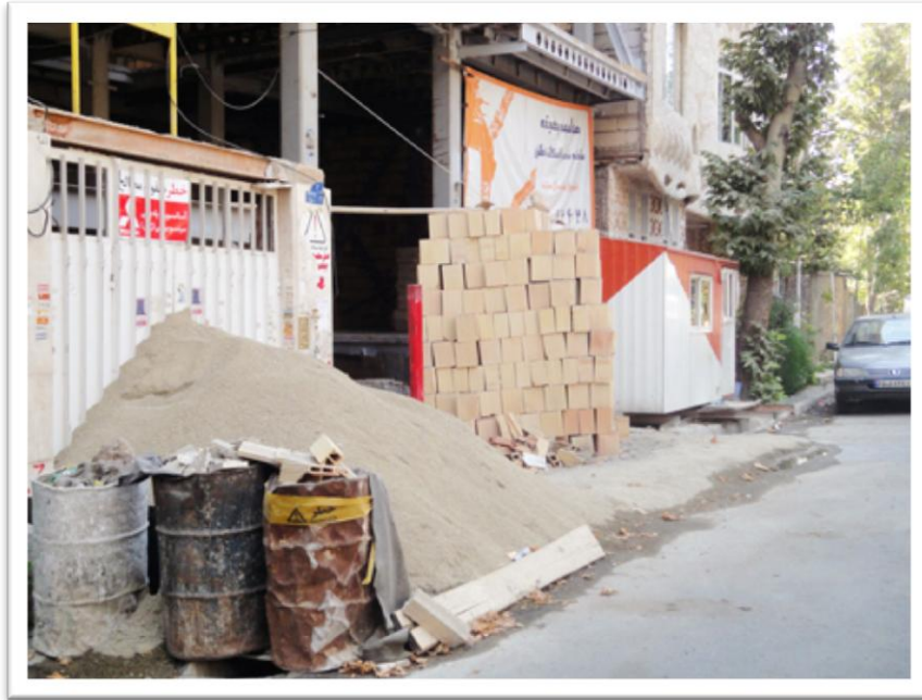
Photo 39: Aggregates and block stored on the pavement
