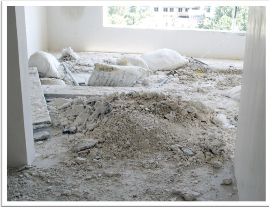
Photo 13: Wasted gypsum powder
