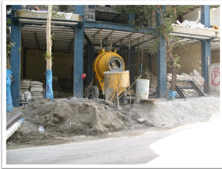
Photo 5: Storing materials in the street in an urban project in Tehran
