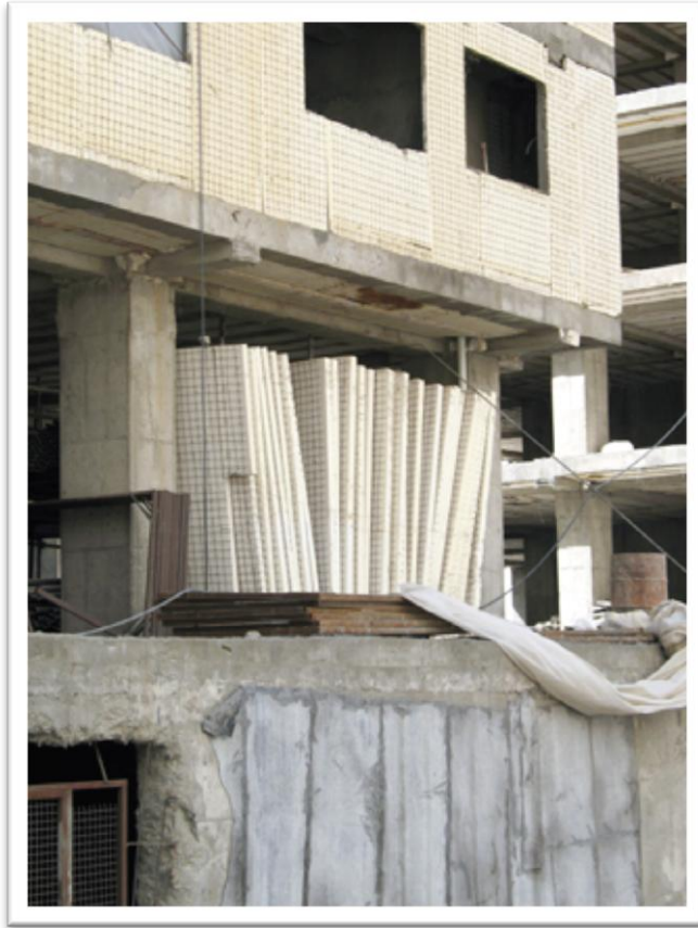
Photo 38: A section in the first floor of the building is dedicated to polystyrene wall units
