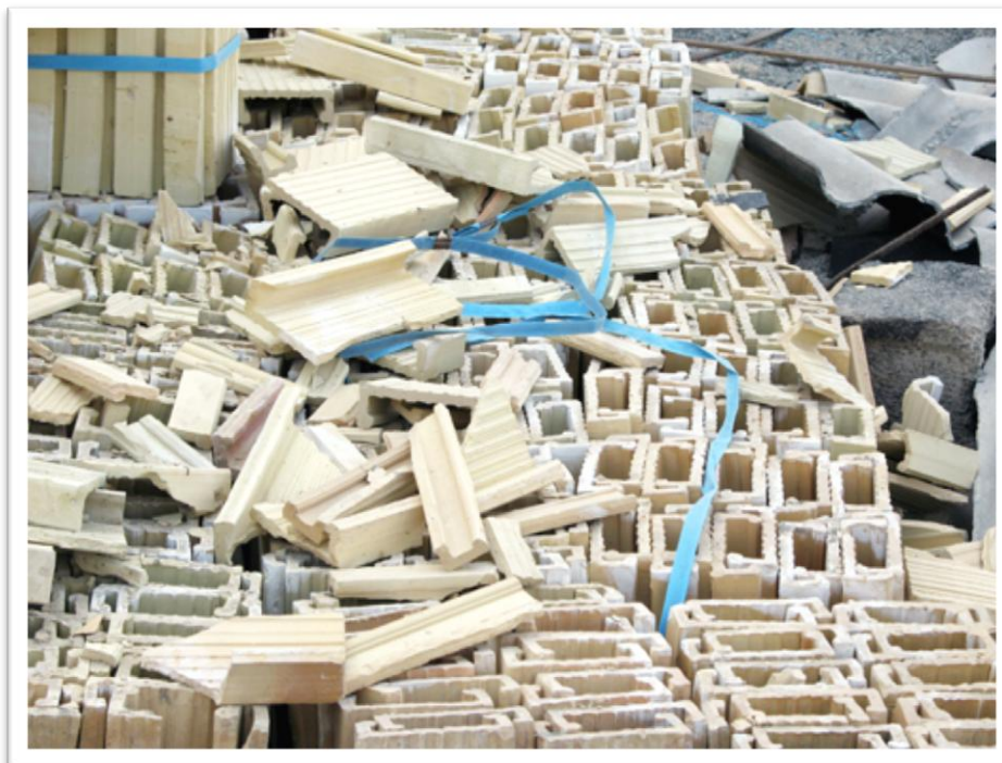
Photo 18: Poor quality packaging of joists' bases
