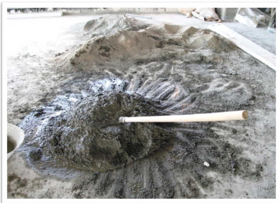
Photo 11: Mixing concrete on floor
