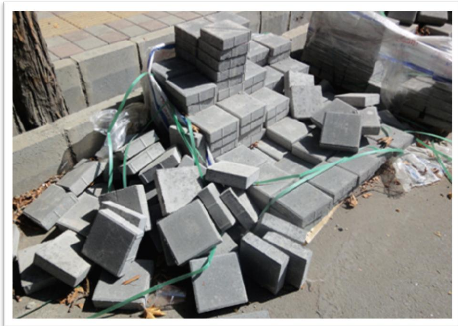
Photo 20: Poor quality packaging of pavement tiles
