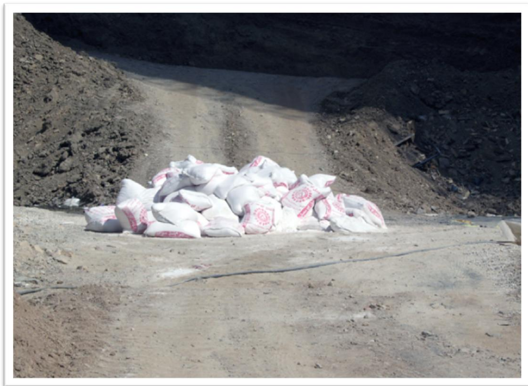
Photo 42: Gypsum powder bags left outside of the onsite warehouse
