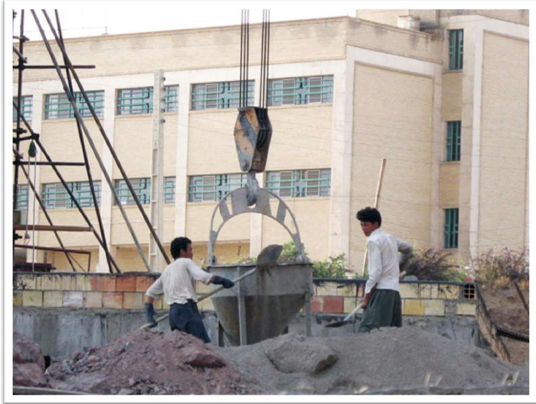
Photo 30: Using a crane bucket to move aggregate to the higher floors
