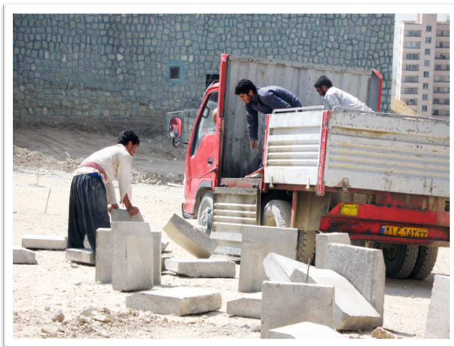
Photo 27: Dangerous unloading of materials (throwing out heavy cement kerbs)
