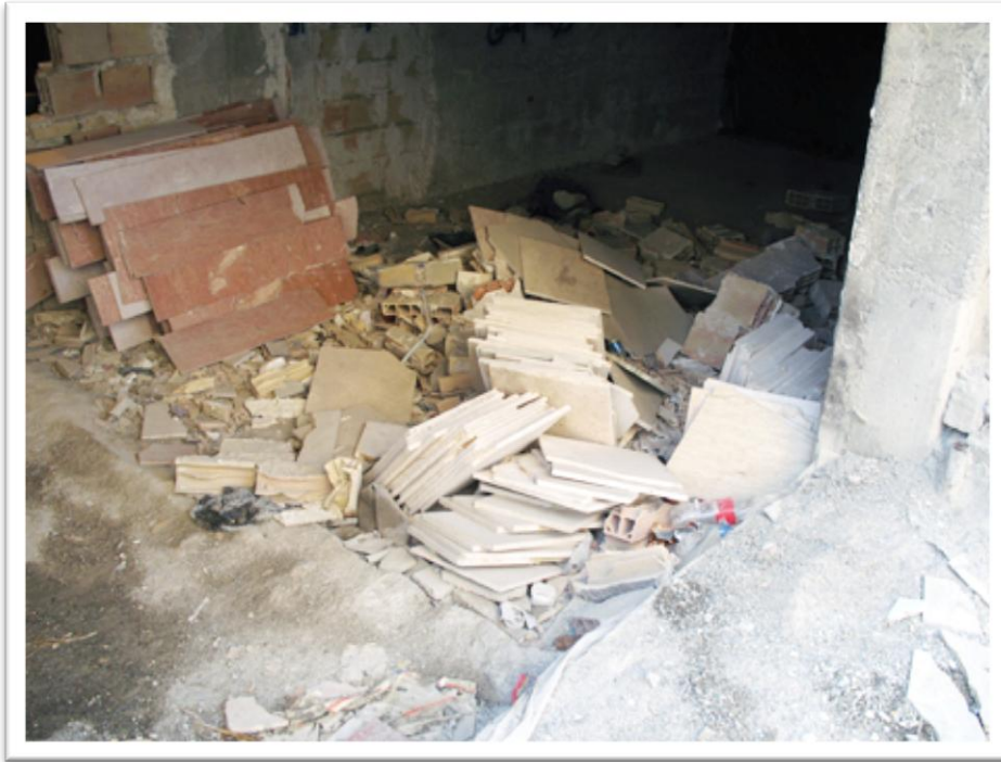
Photo 10: Poor storage of stone
