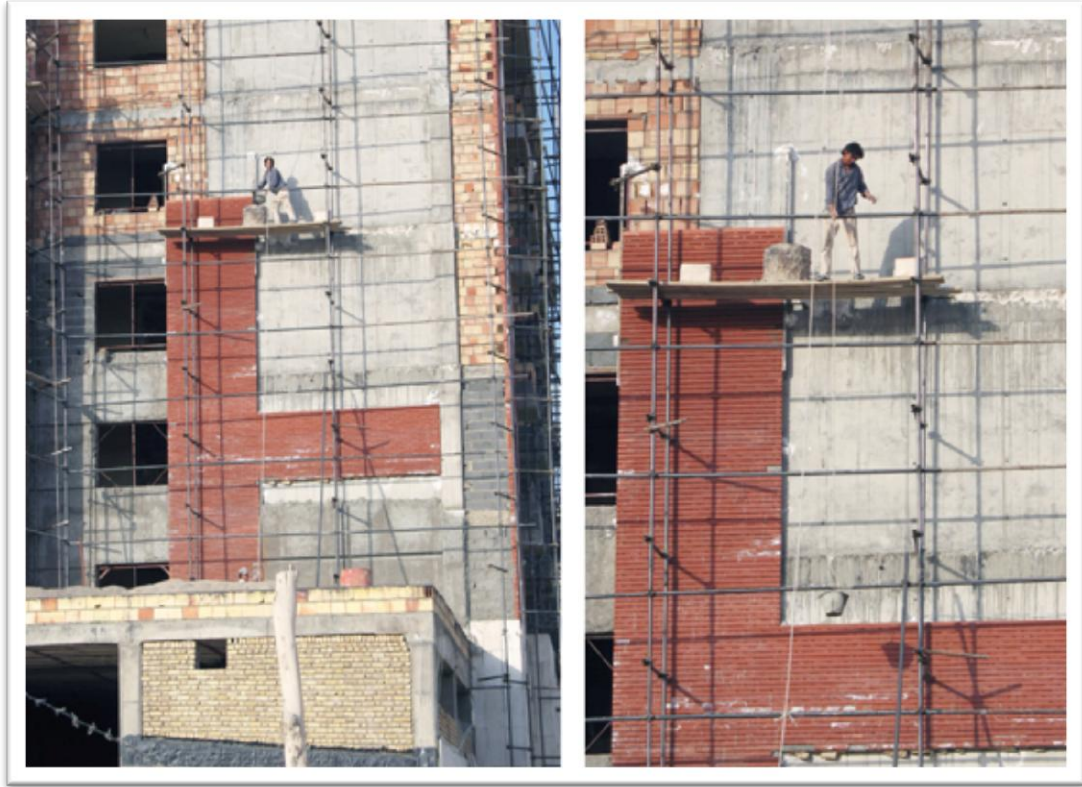
Photo 31: Scaffolds as a risky means for working at height
