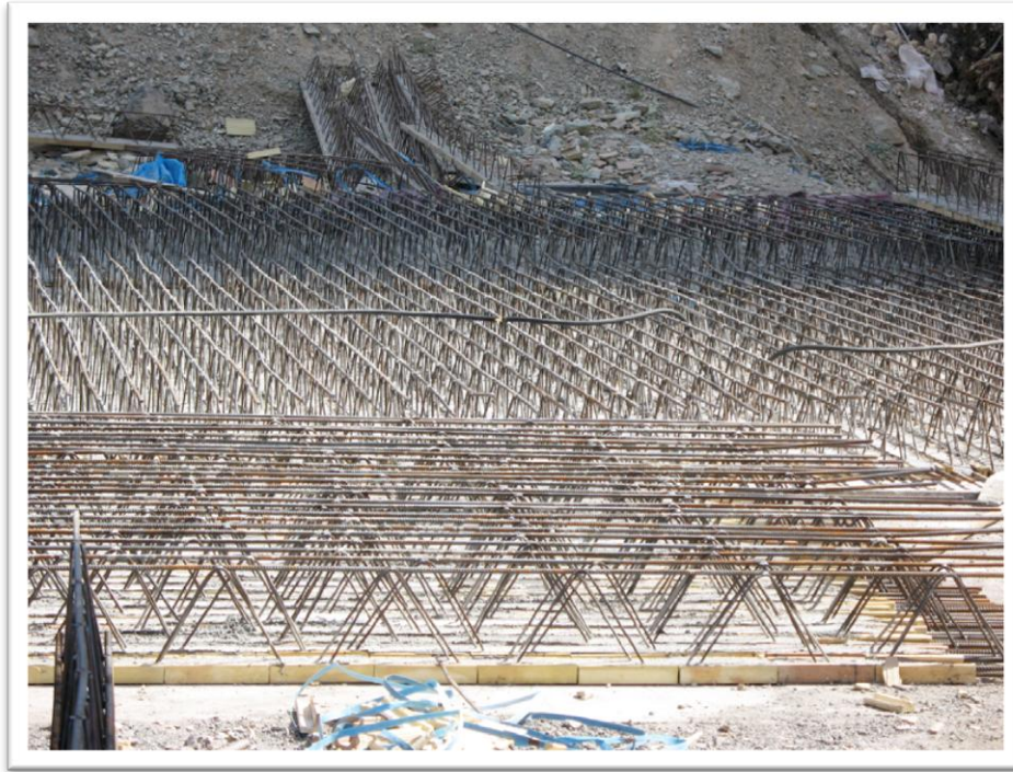
Photo 9: A joist making workshop onsite
