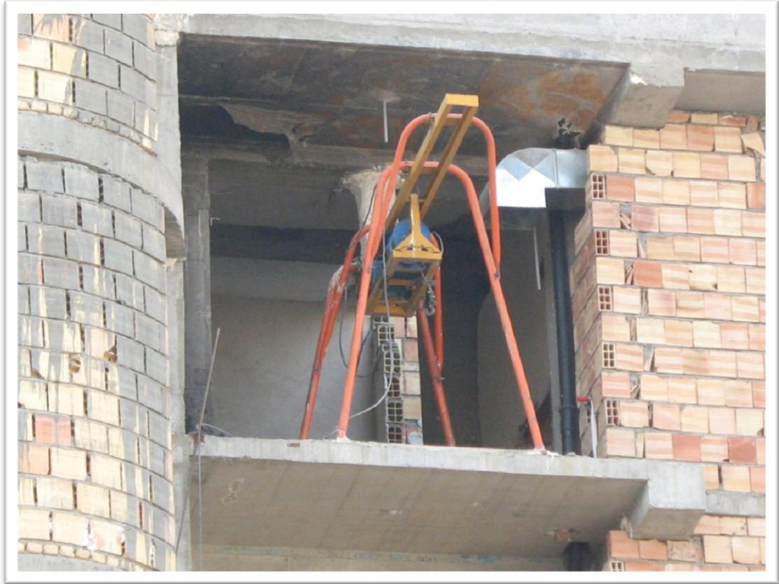
Photo 29: Use of a winch to move materials vertically
