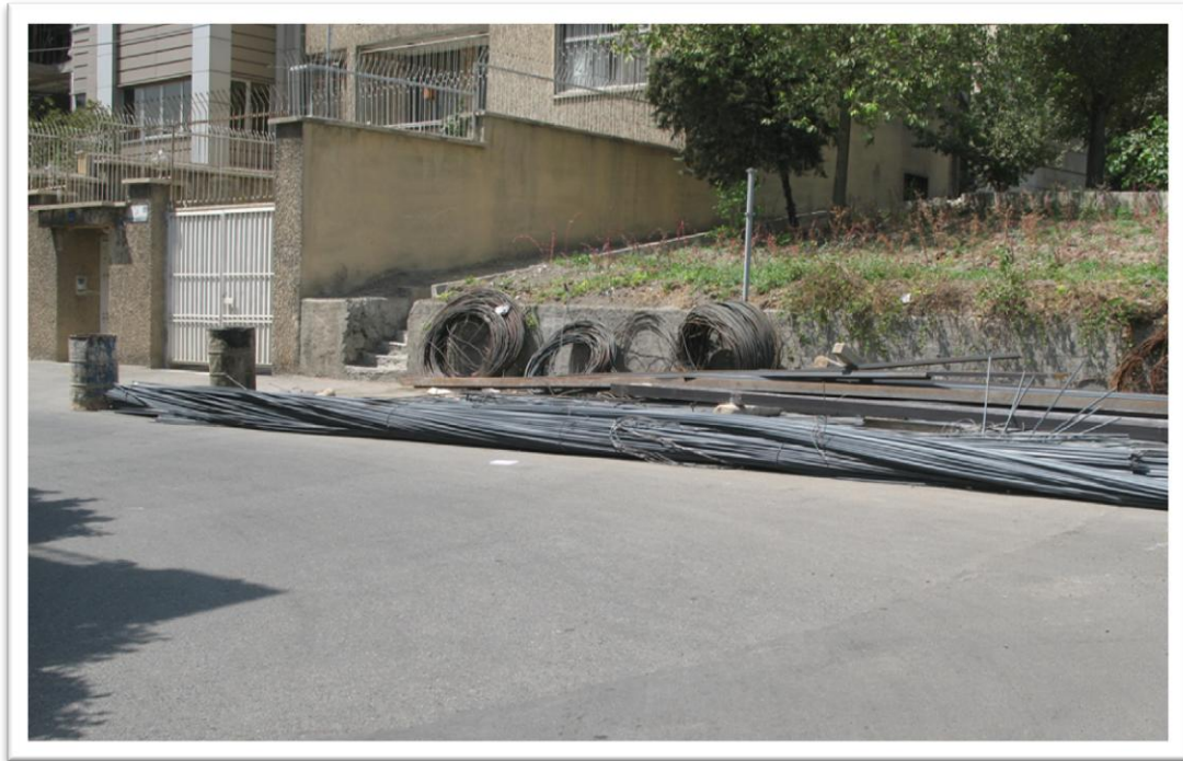
Photo 24: Storing steel rods in the street
