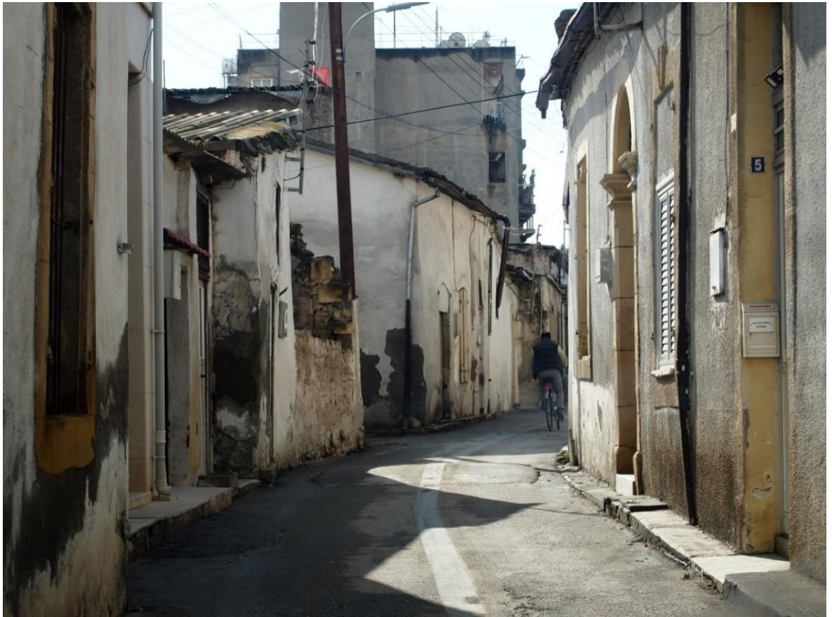
Figure 72: Decaying buildings within the Kafesli/ Yeni Jami area. The light blue line on the street indicates that the area is part of the heritage route created by the NMP as an attempt to encourage people to walk around the historic core and learn about the heritage of walled Nicosia (Author 2016).
