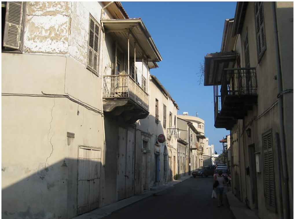
Figure 34: Example of Neglected TC neighbourhood in the South of Cyprus (Author 2013)
