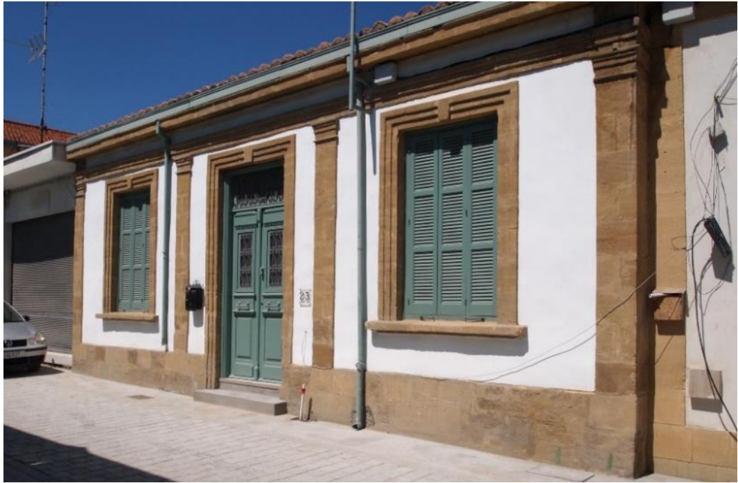
Figure 142 (right): Residential façade restoration in the Chrysaliniotissa area (Author 2014)
