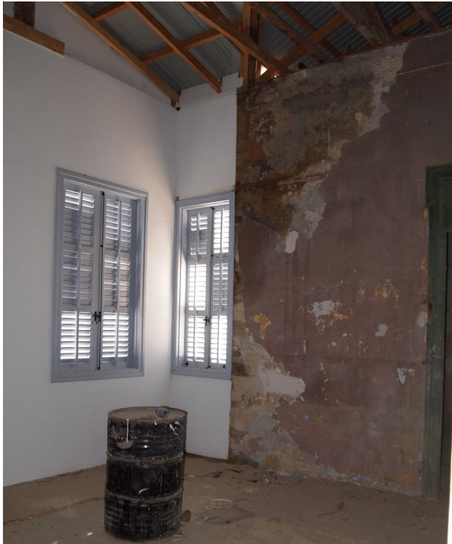
Figure 152: Façade restoration of building located partly in the buffer zone (Author 2017)
