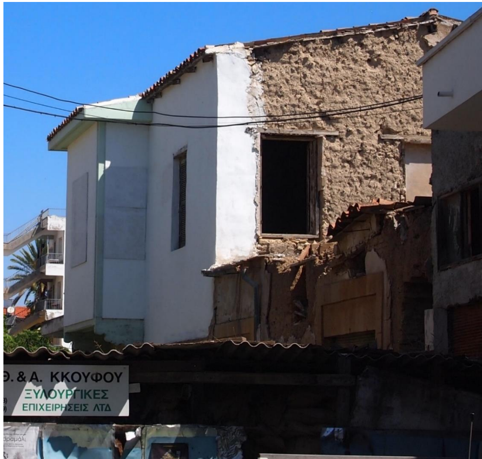
Figure 150: Example of facade restoration in the buffer zone (Author 2014)
