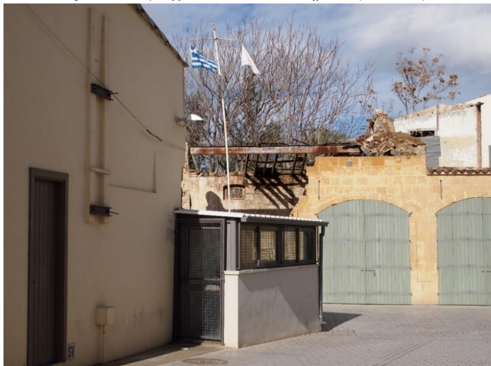
Figure 151: Recently restored building facades, partly in the buffer zone (Author 2017)
