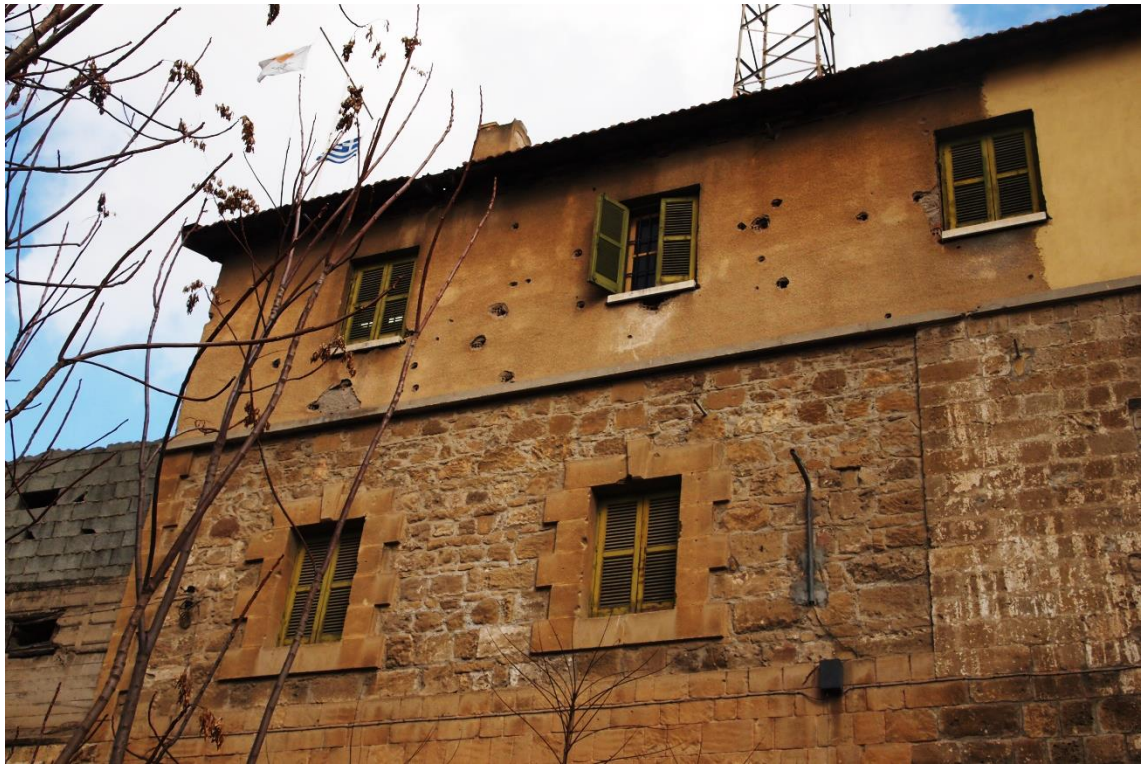
Figure 158: Governmental building (police station) next to the vehicular access and above the pedestrian access of Paphos gate (Author 2014).
