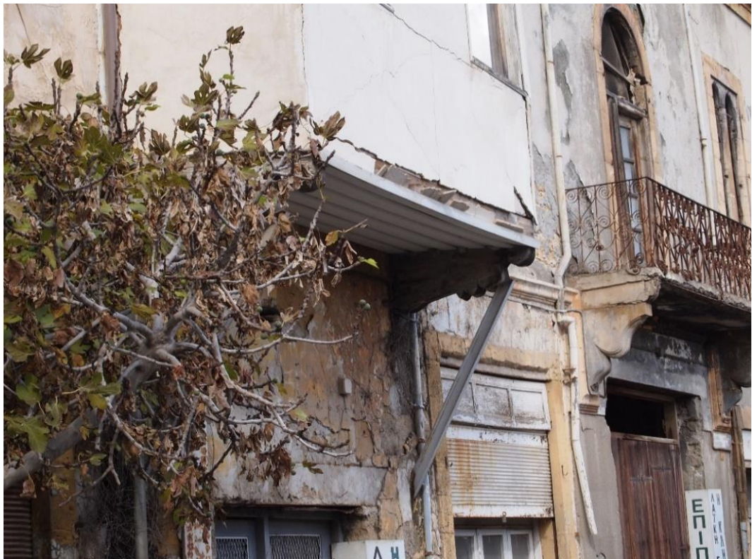
Figure 65: Image illustrating the lack of up-keeping and derelict state of listed buildings in Asklipiou Street (Author 2016). As can be observed, inappropriate propping has been used to ensure the structural integrity of parts of the building that does not comply with local heritage conservation practices. This includes paragraph 1.2b of the Guidelines for the Preservation of Listed Buildings introduced by the Department of Town Planning and Housing (RoC), which sustains that all new interventions need to respect the original fabric of the building, including its material and structural composition (Department of Town Planning and Housing 2008: 4).
