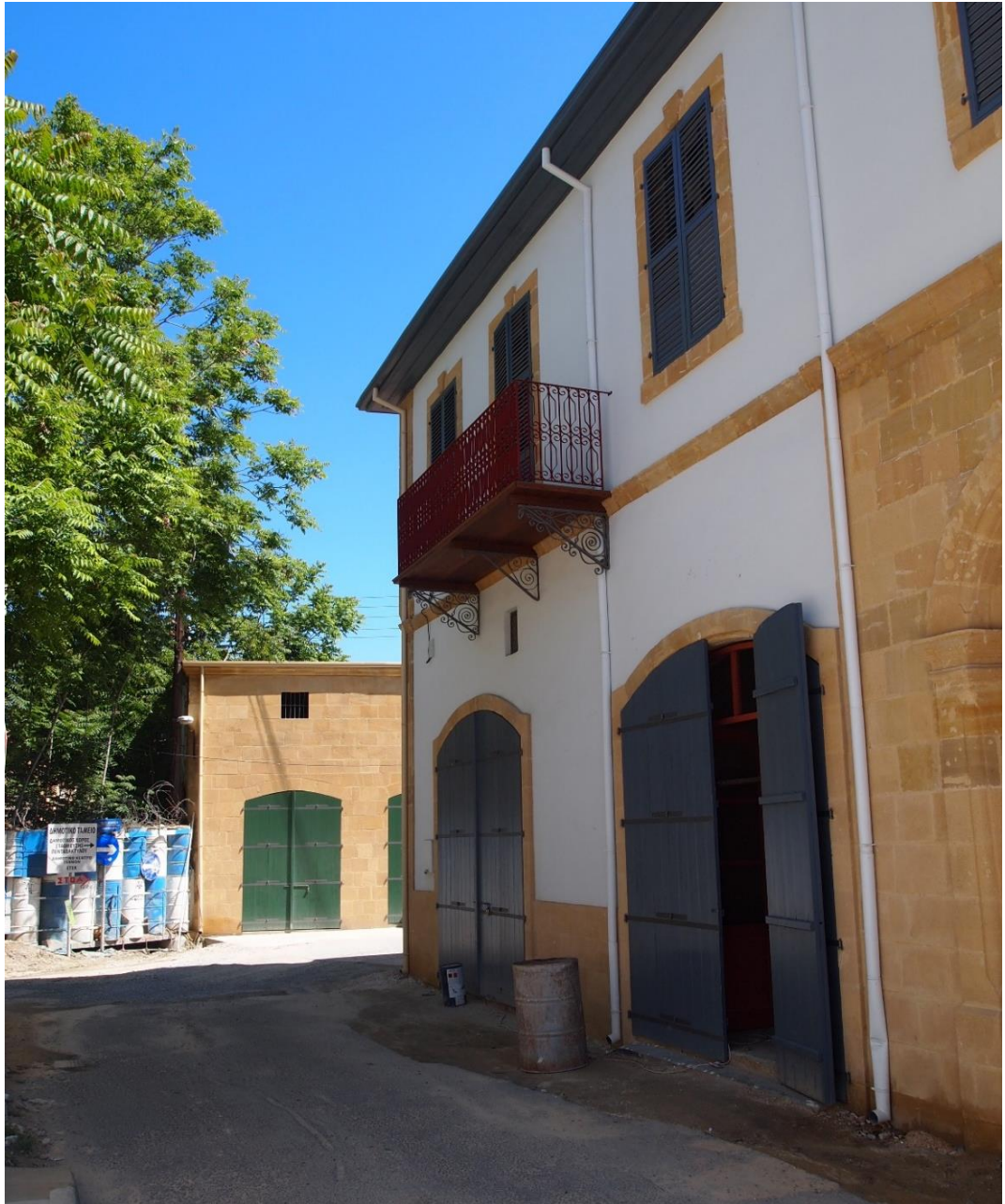
Figure 132: Facade Restoration on Trikoupi Street, adjacent to the buffer zone (Author 2014)
