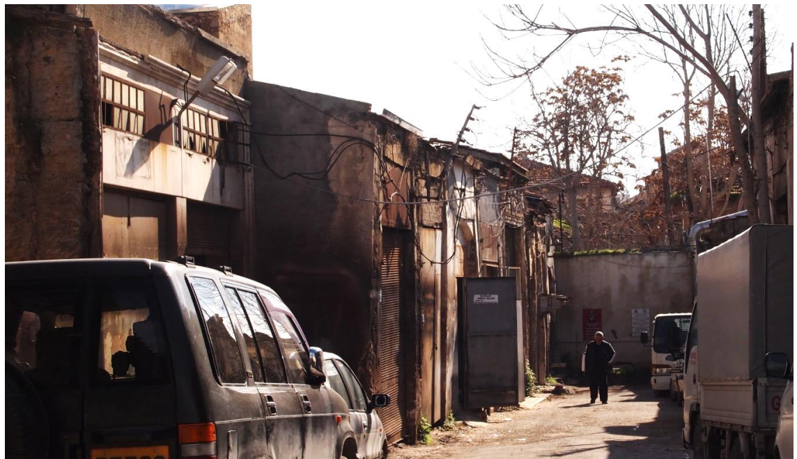
Figure 125: Declining buildings in Selimiye, next to the buffer zone (Author 2012)
