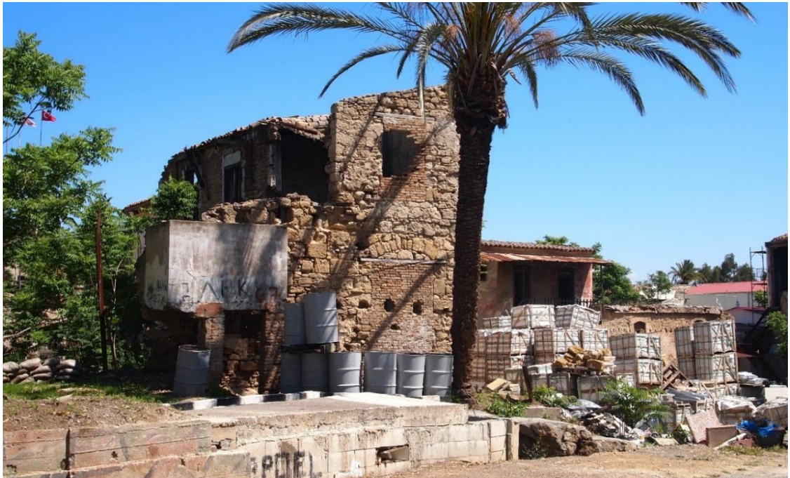
Figure 128: Declining area in Omeriye impacted by the existence of the buffer zone (Author 2014). As can be observed, the site is used as a storage space for construction materials, with surrounding buildings suffering from lack of upkeep and decay.
