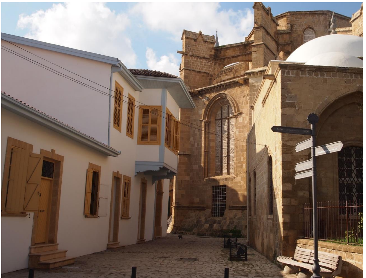
Figure 76: Image of recently restored building in the Selimiye area (Author 2012).
