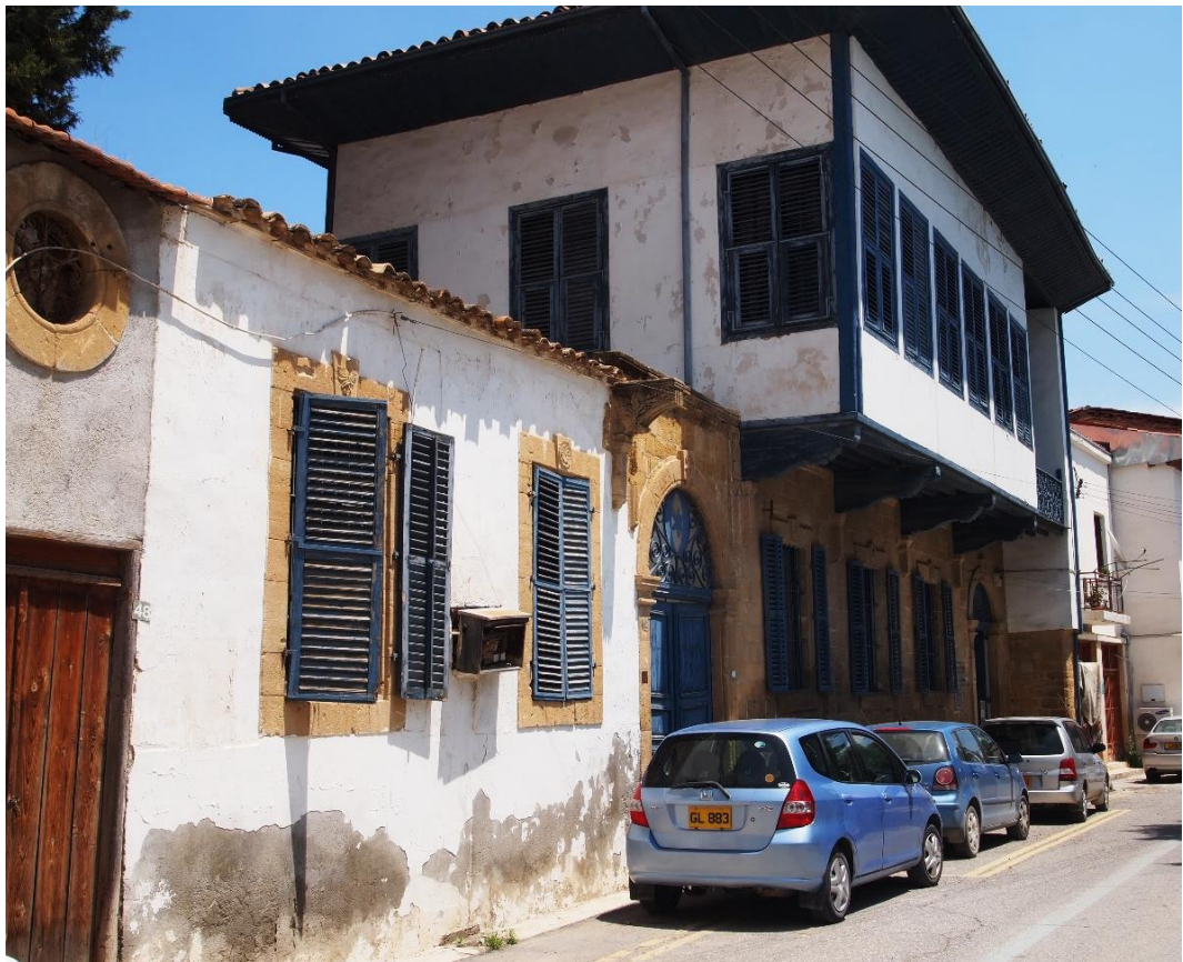
Figure 143: Restored building in Arab Ahmet showing signs of a lack of maintenance. This building was previously restored as part of the NMP initiative (Author 2014)
