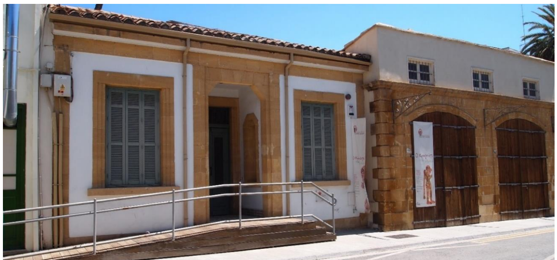
Figure 16: Buildings on Ektoros Street have also been adopted to suit contemporary needs (in this case a museum) (Author 2014)
