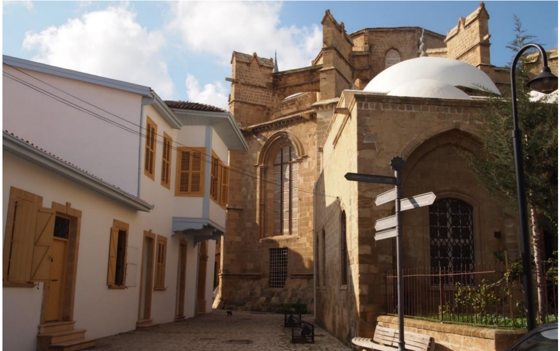
Figure 134: Example of building rehabilitation on the south side of Selimiye mosque (Author 2012)
