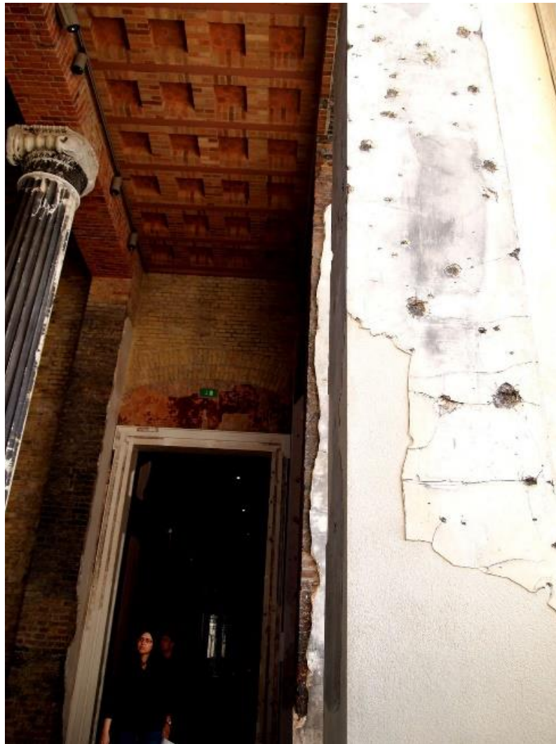
Figure 47: Details from the restored Neues Museum (Author 2011)
