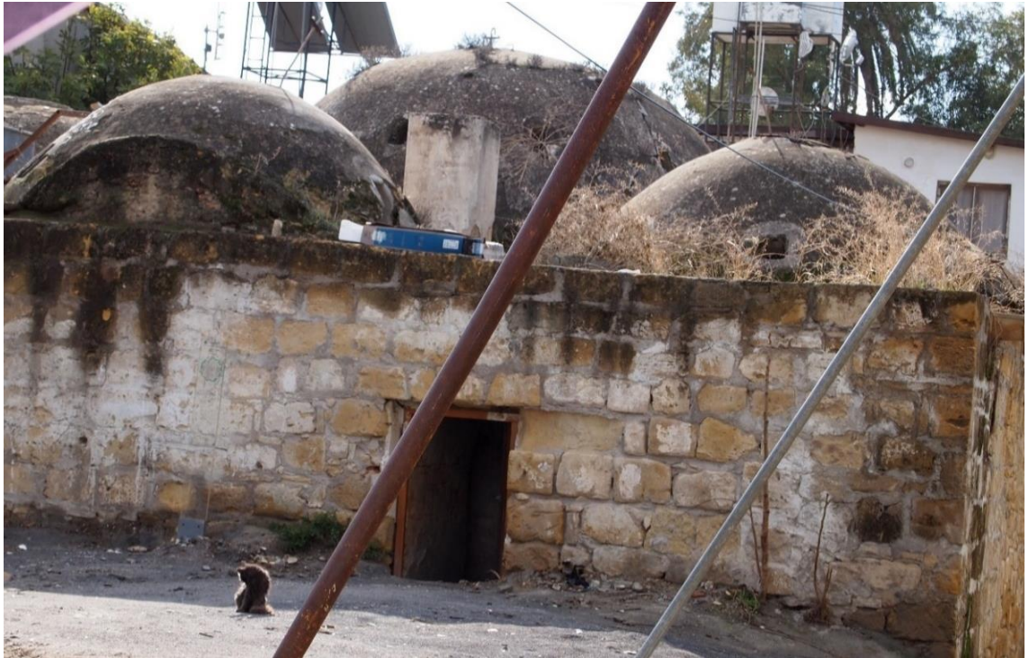
Figure 73: Decaying building within the Kafesli/ Yeni Jami area. Image of Tandi's Hamam, left to decay since the division of the city, where materials were removed to be used for the construction of military posts (Author 2016).
