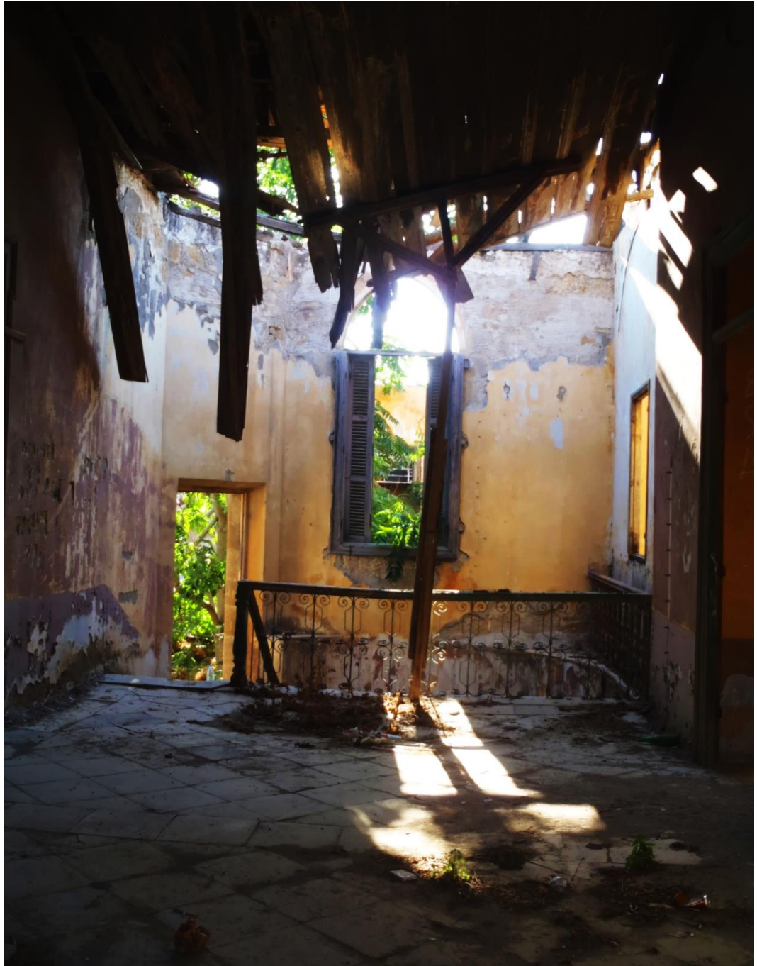
Figure 68: Image illustrating the first floor of the same residence presented in Figure 67 (Author 2012). As can be observed, the roof of the building has collapsed, consequently preventing any protection from the elements, while encouraging its accelerated structural decay.
