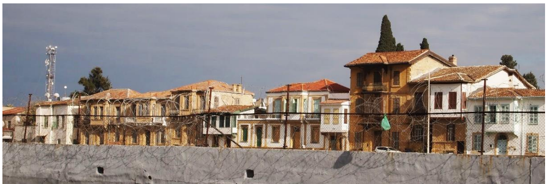
Figure 137: Zahra Sokak residences at the east edge of Arab Ahmet (Author 2017)
