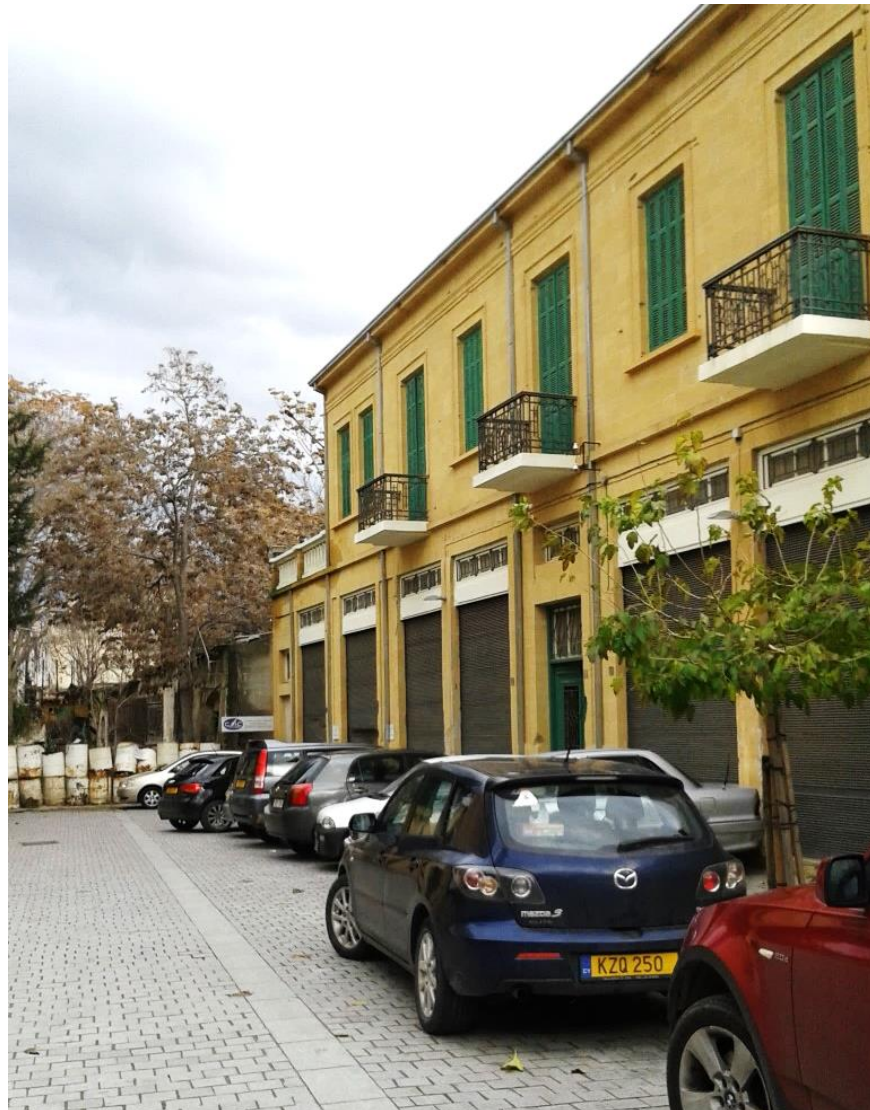
Figure 162: Recently restored building facades on Paphos Street, walled Nicosia (Author 2017)
