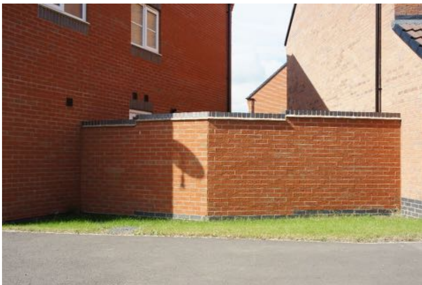
Figure 57: Dead space. Here a potentially pleasant sunny spot that could help to enliven the street and create an enjoyable place for residents is instead a patch of ground that will become forgotten and neglected (10. Saxon Gate). 2013.
