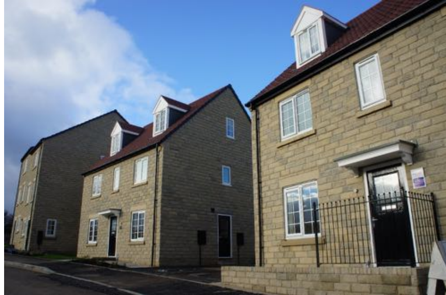
Figure 36: The use of local stone to the facades of standard house types makes a marked difference to creating place with a sense of locally inspired character (8. Weavers Gardens). 2013.
