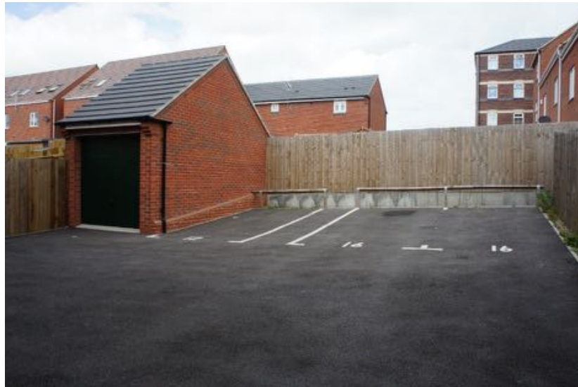
Figure 52: A typical parking court - unlit, lacking surveillance and dominated by hard materials (3. Briars Chase). 2013.
