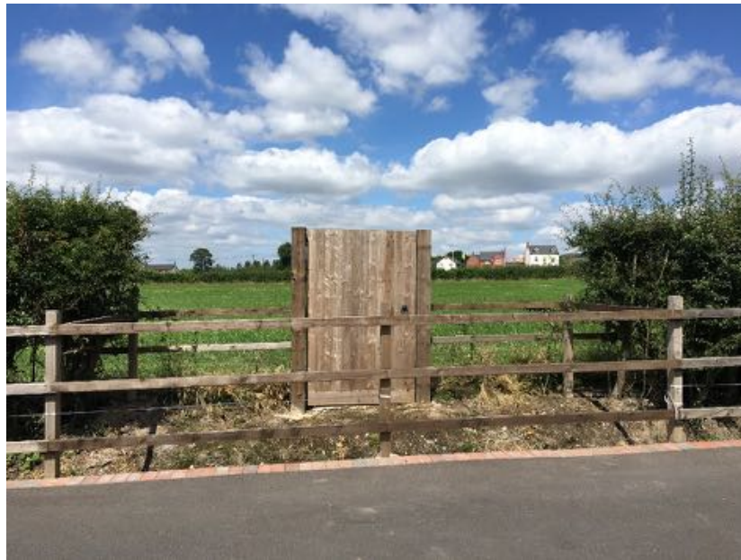
Figure 104: The requirement for a field gate to allow agricultural vehicle access to the field beyond was misinterpreted by the contractor following the two-dimensional boundaries plan. Ashby de la Zouch. 2017.
