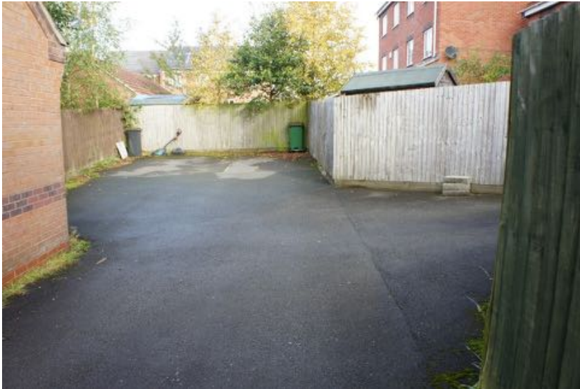
Figure 124: A poorly overlooked car parking courtyard. Note the poor level of general maintenance, lack of lighting, abandoned building materials and garden equipment. The plan extract (Figure 125) shows this courtyard behind the rear of plots 46-49. Note the distinct lack of landscaping within the courtyard compared to the clear suggestion of generous tree planting within this space.
