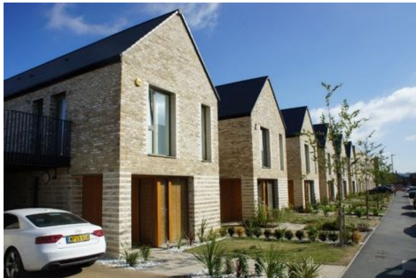
Figure 86: New streets at Edgware Green in London (Barratt Homes) demonstrate that organic inspired design is not the only way to deliver well designed streets and developments. 2016.
