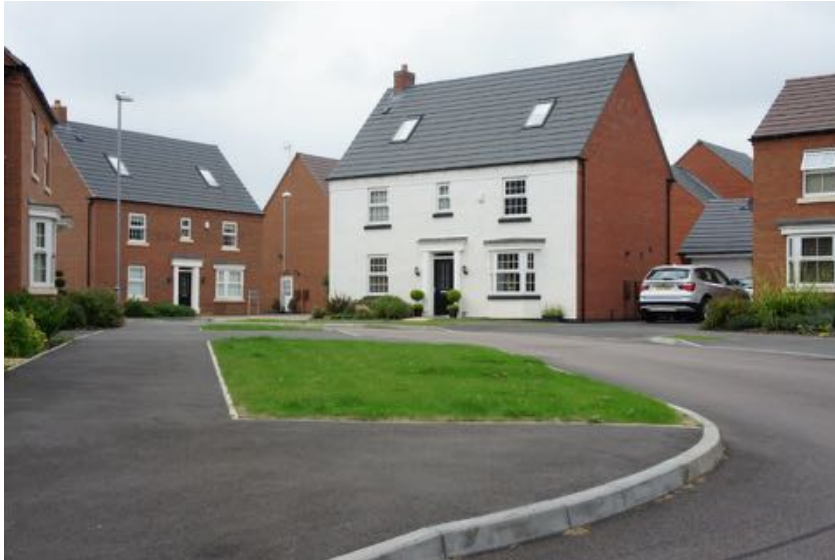
Figure 41: Organic inspired schemes were often compromised by over-engineered highways designs. Features imposed on developments by highways authorities typically include forward visibility splays that across a development can consume a large amount of space. It is not uncommon for these areas to be used as informal parking spaces. 2013.
