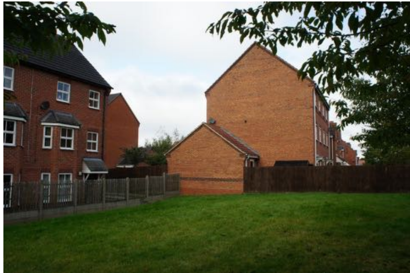
Figure 123: The poor relationship between buildings and open spaces is evidence to two dimensional 'plotting' as opposed to three-dimensional thinking about how buildings and spaces work. Please cross reference image to the 'play space' towards the bottom and centre of the layout plan shown in Figure 122.
