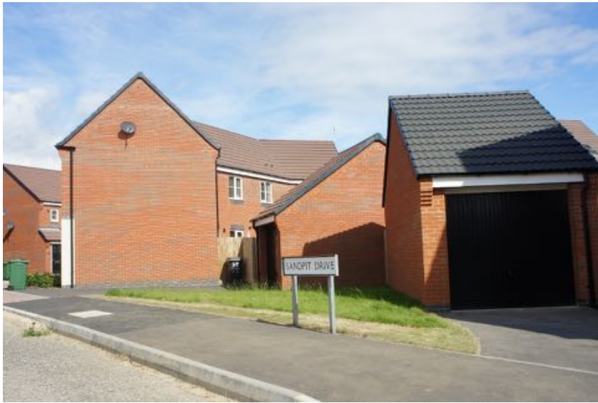
Figure 45: A fragmented and uncoordinated building arrangement creates wasted spaces with no clear public or private function. (14. Jasmine Gardens). 2013.
