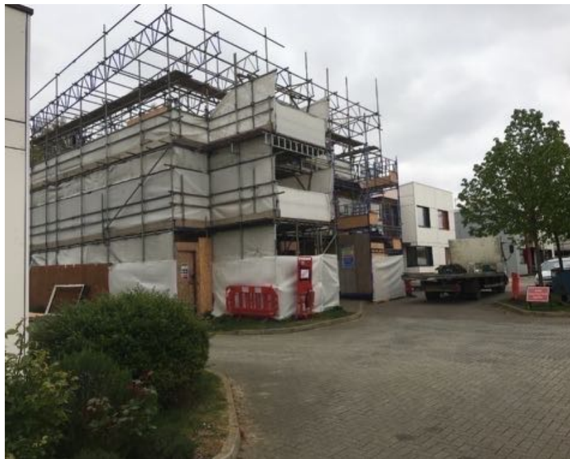
Figure 32: Oxley Woods . The Building for Life Award winning, Manser medal winning and “critically acclaimed quick-build housing system” 81 pioneered at Oxley Woods, Milton Keynes by Richard Rogers was the flagship of John Prescott’s Design for Manufacture competition: low cost, low energy homes showcasing off-site manufacturing techniques. Some homes are currently being repaired with parts of the timber frame being repaired or replaced. Homes are being afforded a new construction detail to safeguard against future water egress. Milton Keynes. 2016.
