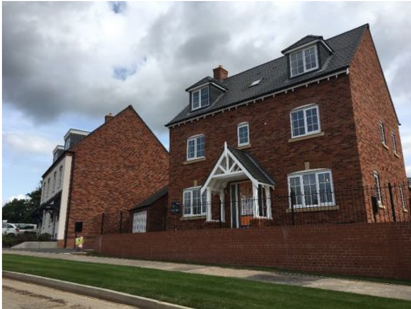
Figure 103: Changes in carriageway levels resulted in the street ‘dropping’ creating an unforeseen level change between the back of the pavement and the front door. Whilst the developer secured consent for the changes in carriageway levels from the highways authority (County Council), they failed to notify the planning authority (District Council). A potential breach of planning is now being investigated. Whatever the outcome, the finished development will not be as envisaged as the planning authority does not consider it has a strong enough case to require this particular house to be rebuilt level with the street partly on the basis that Permitted Development Rights were not removed. If site staff had access to augmented reality the risk of deviating from approved (multiple) plans could have been identified prior to the laying of foundations. Ashby de la Zouch. 2017.
