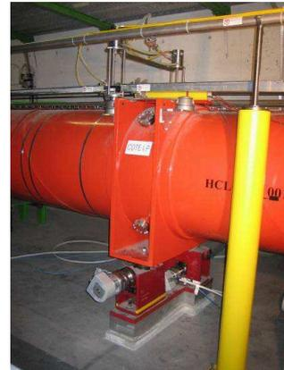
Fig. 2: Sensors and motors installed on a low beta quadrupole
