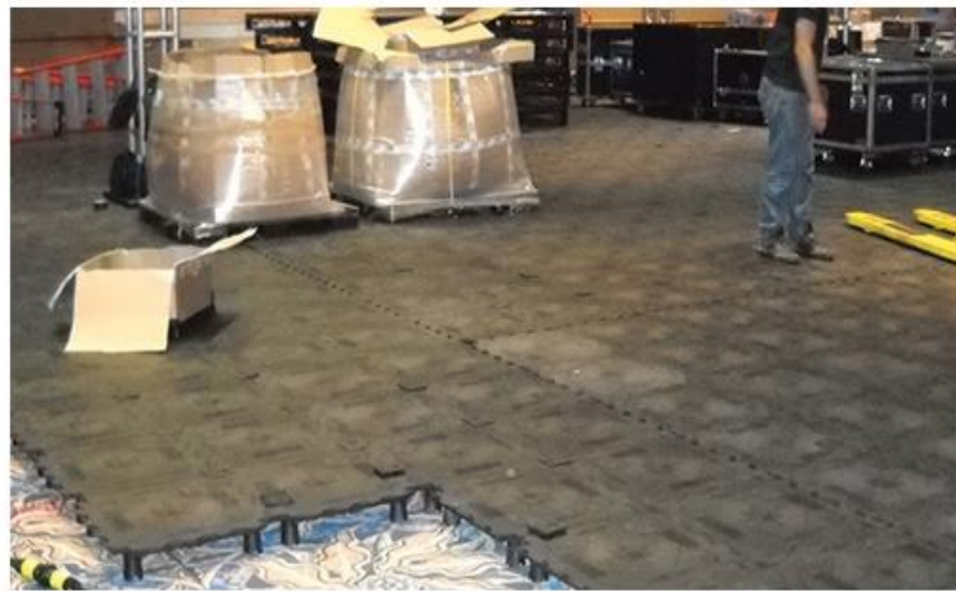
Figure 7.4 Plastic low profile raised floor panel (EFS, 2015a, b)
