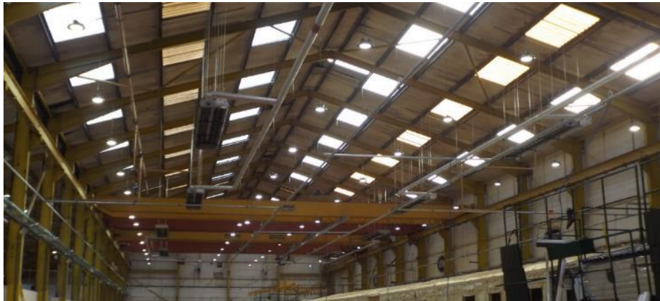
Figure 4.1 Industrial LED lighting application scenario.
