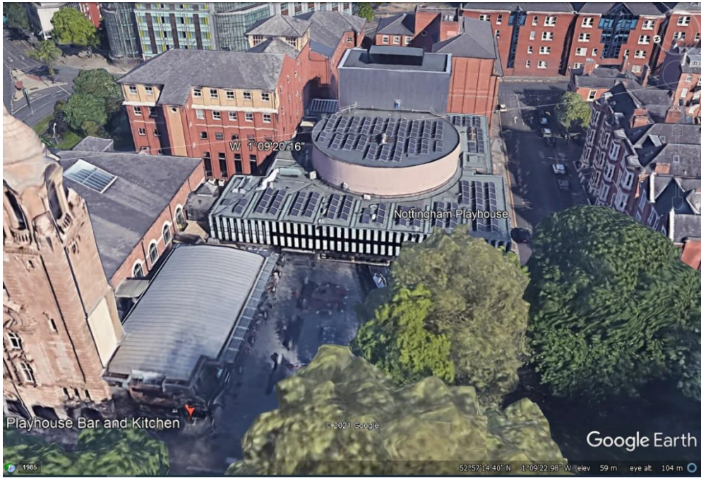
Figure 25: Post-retrofit Nottingham Playhouse with the photovoltaic solar panels on the roof (Credit: Google Earth, under Geo Guidelines ).
