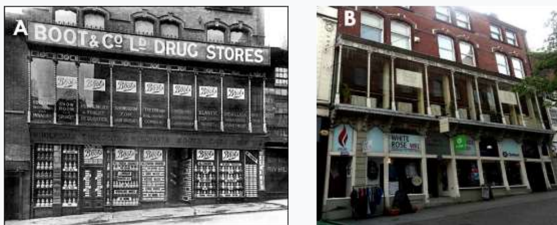
Figure 6.2: A: The first Boots shop, Goose Gate (1885). Source: Clapp (2013). B: The building today. Source: Almakkas, 2018
