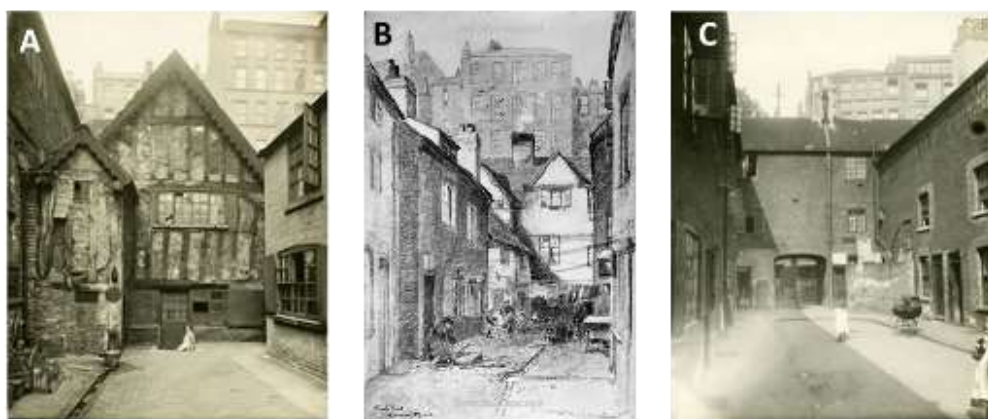
Figure 4.10: Poorly built and lacking sanitation and basic facilities
