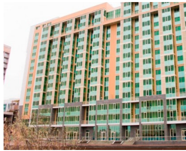
Figure 3. Comfort class building.
