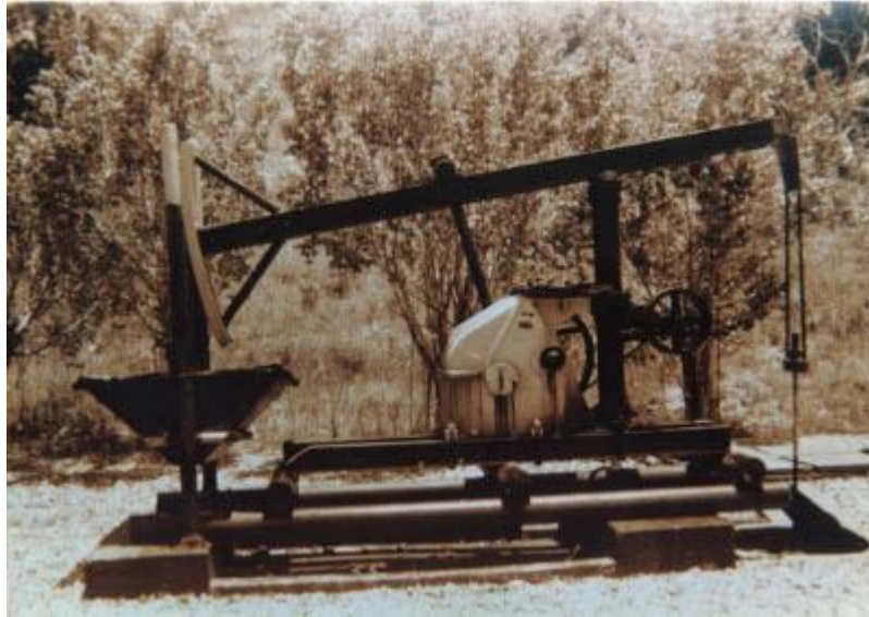
Photo 1: Tropical Oil Company oil well (Tapias Cote, 2012).
