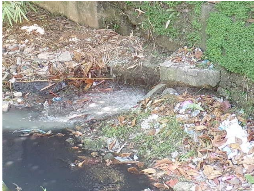
Photo 3: point of discharge of an informal sewage pipe in the neighbourhood of Arenal, comuna 1 (04/05/2018). The water is discharged in an open canal that receives waste from other dwellings within the area.
