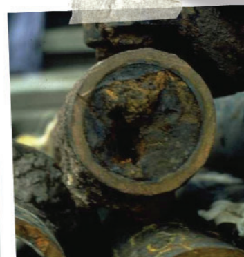
The state of some existing water pipes
