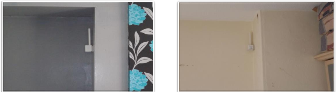
Figure 3.3: Sensors measuring room temperature
