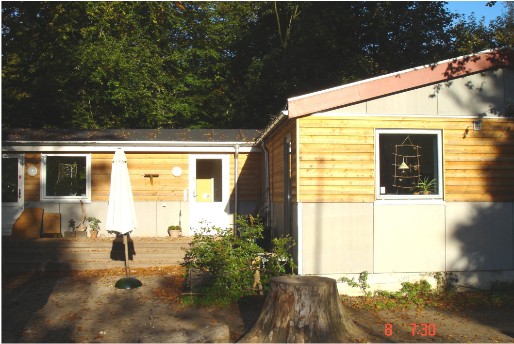
Illustration 4 The Danish nursery building
