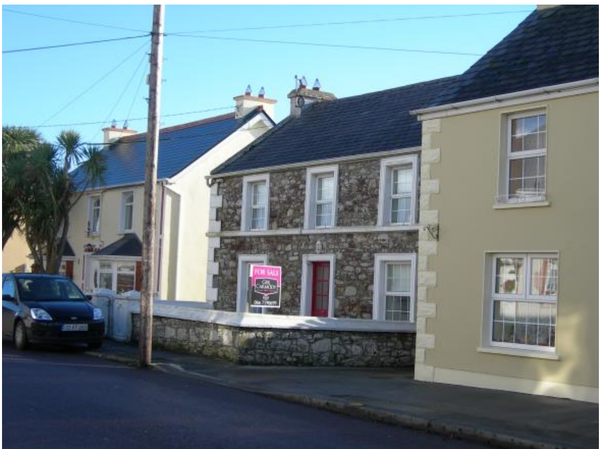
Image 21: 19 th century building with render removed to expose random rubble substrate, Ballyheigue, County Kerry. (Photographic credit: Ramona Usher)
