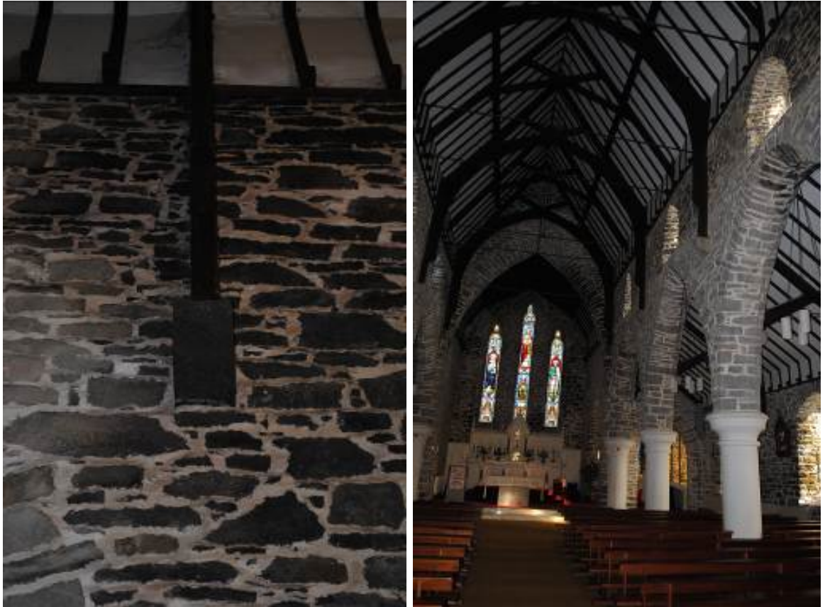
Image 17 and 18: St Brendan's Church, County Kerry. Internal plasterwork removed. (Photographic credit: Ramona Usher)
