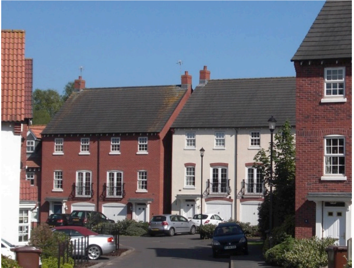
Image 25: New housing development, Mount Sorrell, Leicestershire, UK. Chimney stacks in centre are rotating. (Photographic credit: Tim Peach)
